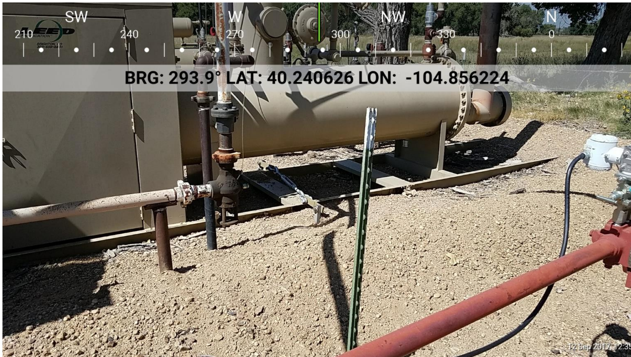
Flood Anchoring on Separator COGCC Location Number: 329974
