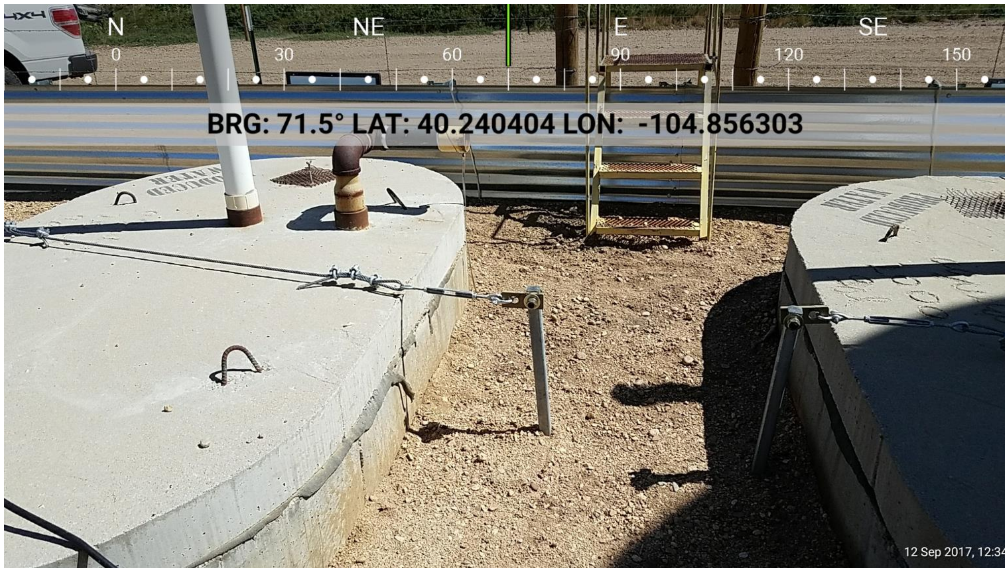
Produced Water Vault Flood Anchoring COGCC Location Number: 329974
