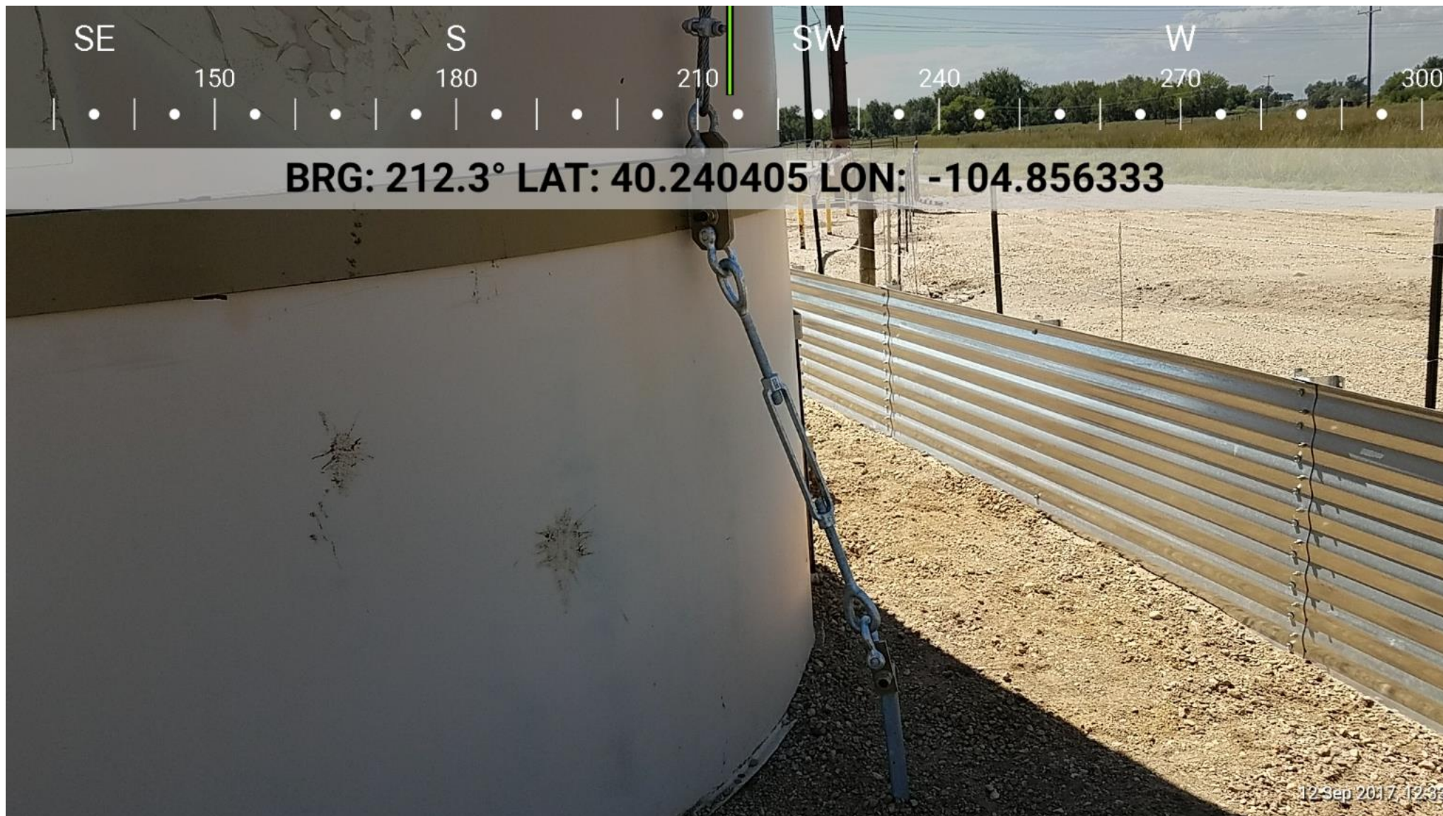
Flood Anchor on Crude Oil Tank
