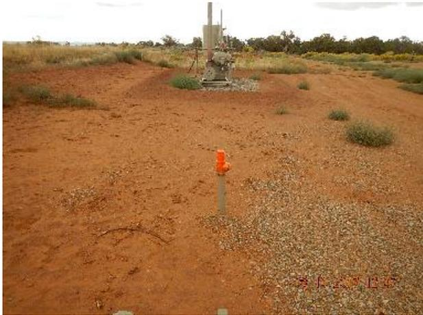
**Photo 11: Unused riser between separator and gas meter shed.**
