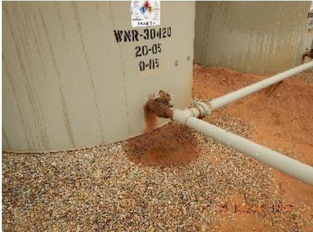
**Photo 5: Impacted soil below tank valve.**
