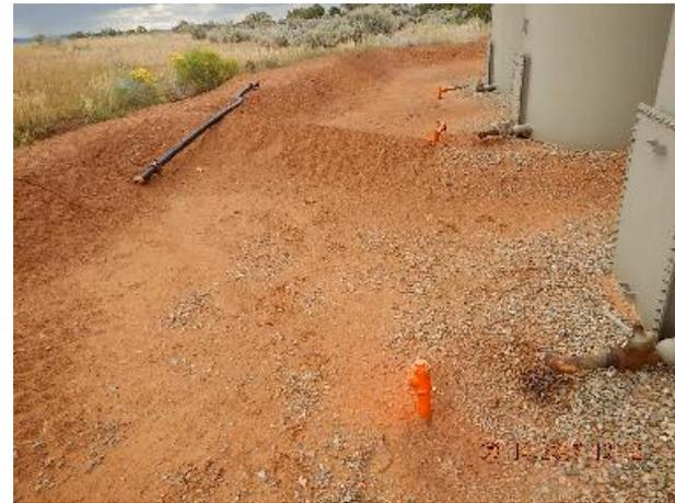
**Photo 8: Pipe section and unused risers inside berms of production tanks.**
