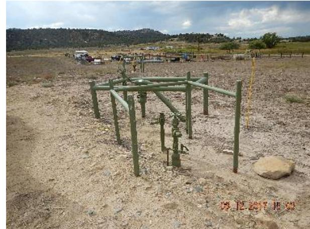
Photo 8: Group of (3) steel risers N side of meter run shed.
