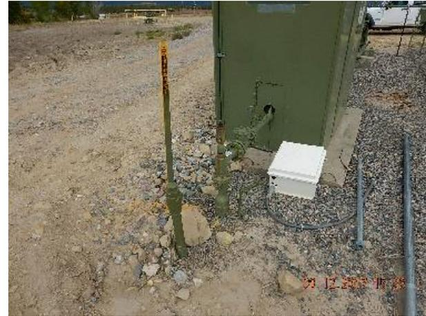
**Photo 10: Unused risers on W side of meter run shed.**
