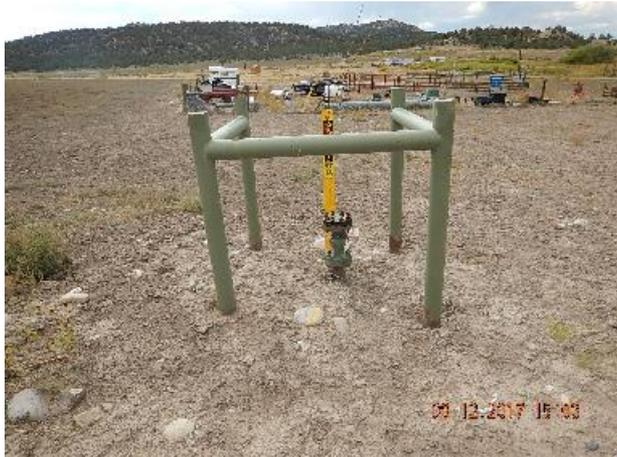
Photo 7: 4" steel riser NW of gas meter run shed .
