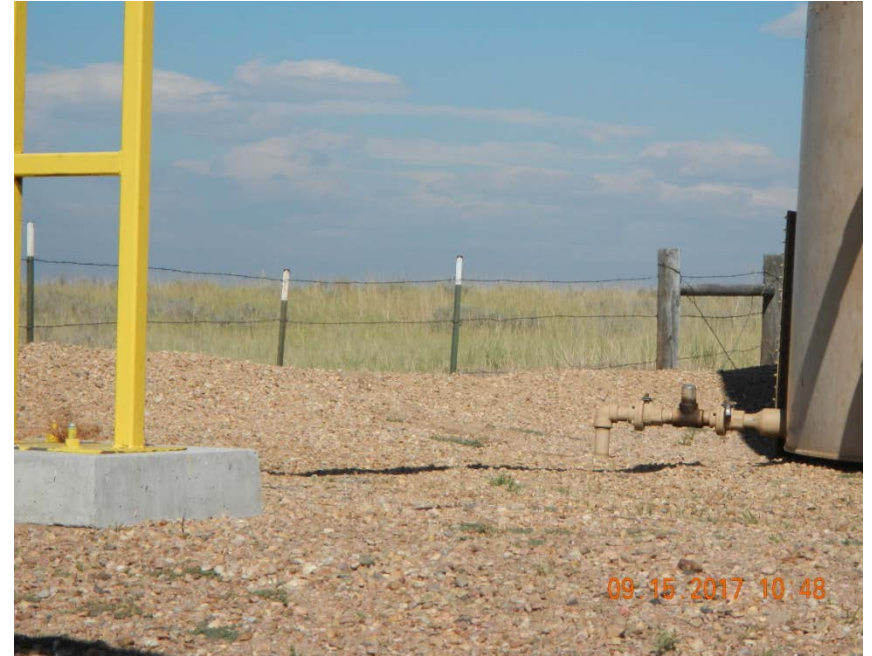
Crude oil tank berm
