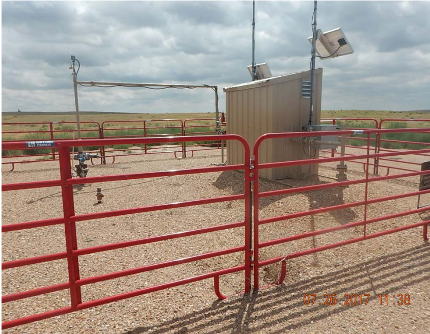
Photo 1: Wellhead, looking SE
