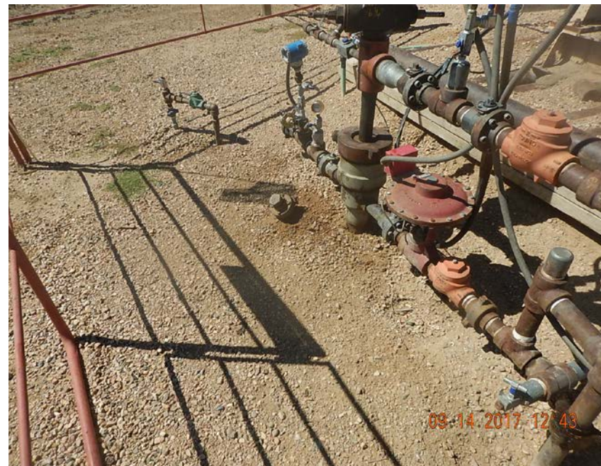
Photo 4: Stained soil at wellhead.
