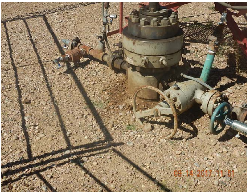
Photo 3: Stained soil at wellhead
