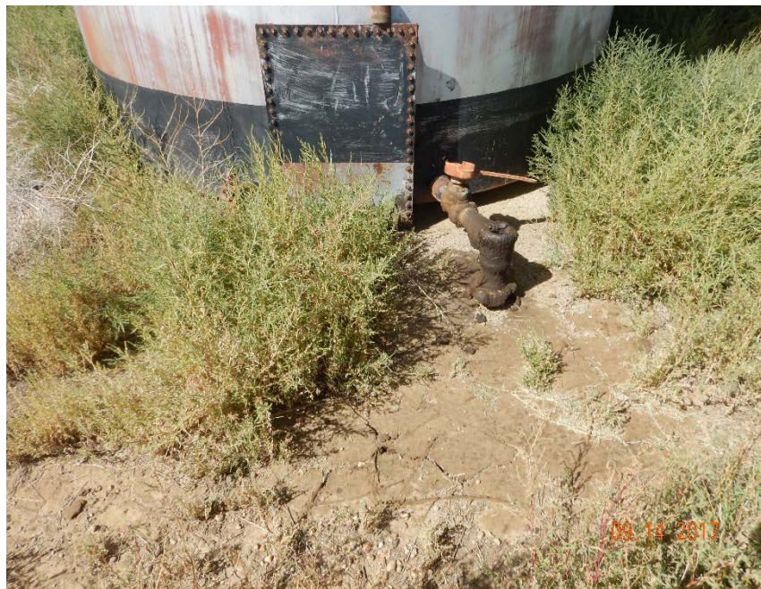
Photo #3 – Historical accumulation of oily waste beneath crude oil AST valve.
