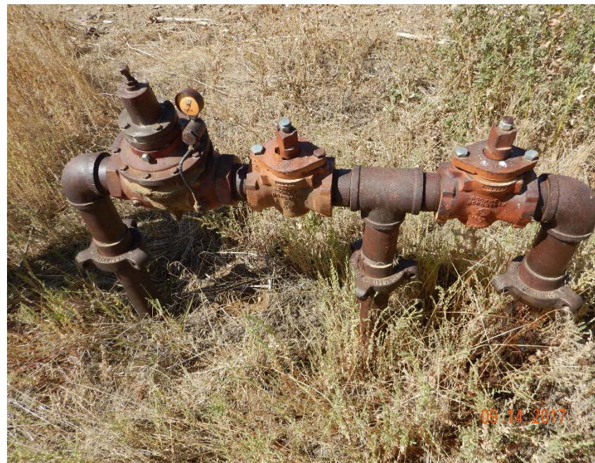
Photo #8 – Second exposed flowline riser manifold located north of equipment in previous photo. Note: 3" pipe on the right is uncapped and facing downward.
