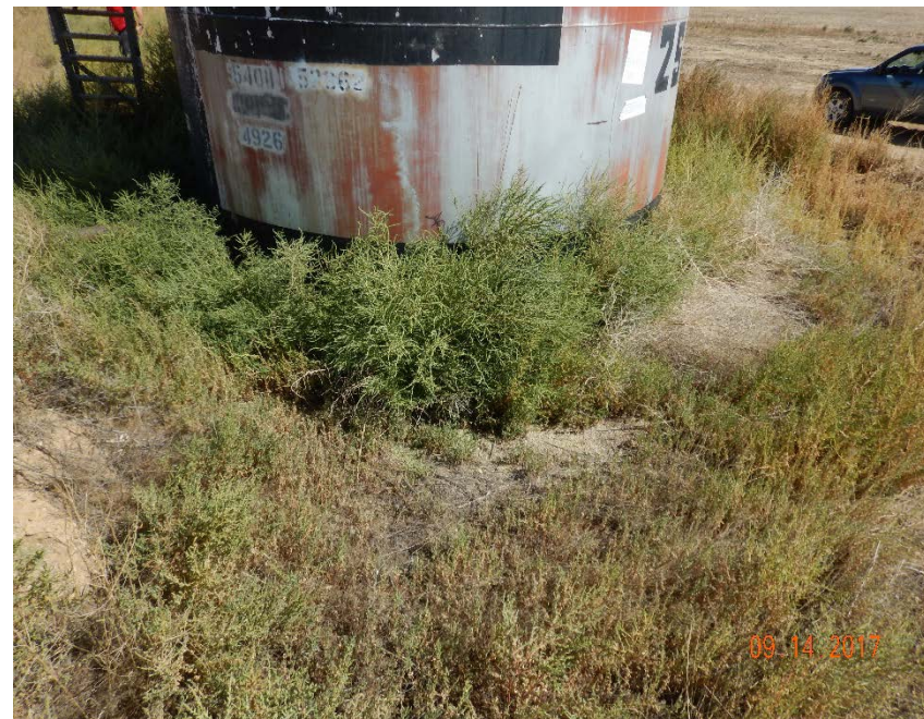
Photo #2 – Uncontrolled weeds inside of tank berm.
