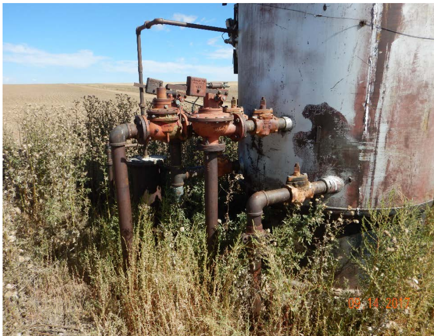
Photo #9 – Unused flowline risers plumbed to VHT on north side of production facility.
