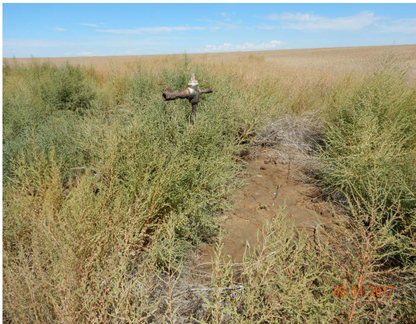
Photo #11 – Schmidt #1-B wellhead with localized accumulation of oily waste and uncontrolled weeds.
