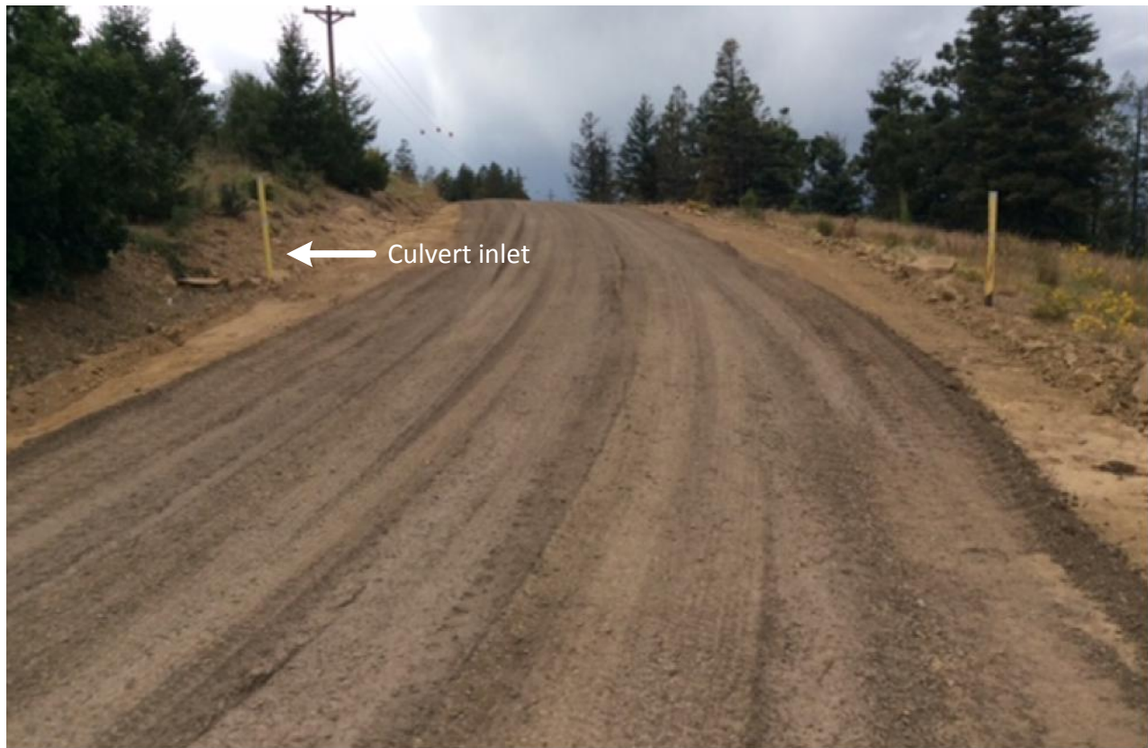
Photo 1: Facing west along the main access road. Installed road base and crowned the driving surface to establish sheet flow. Dominated the bar ditch to direct run off to the culvert inlet.
