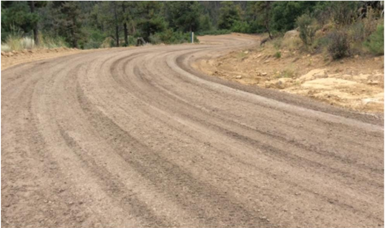
Photo 3: Facing further down the road to the southeast. Installed road base and crowned the driving surface to establish sheet flow. Dominated the bar ditch to receive run off.
