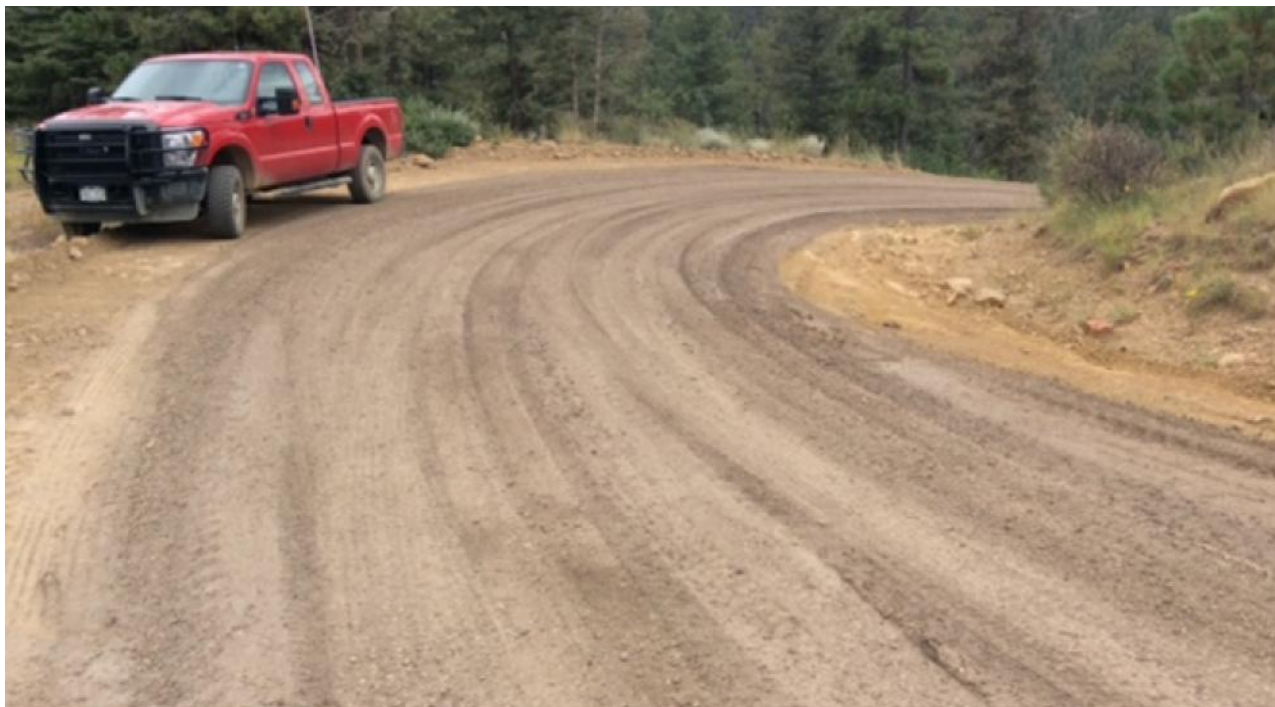
Photo 2: Facing down the road. Installed road base and crowned the driving surface to establish sheet flow. Dominated the bar ditch to receive run off.
