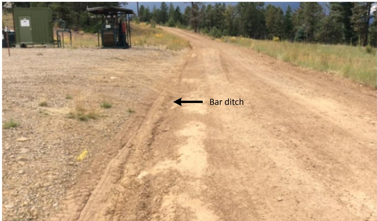
Photo 5: Facing west along the main access road adjacent to the well pad. Dominated the bar ditch to receive run off.
