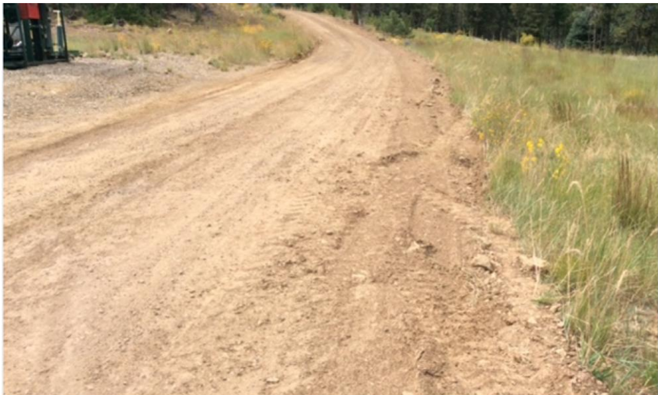
Photo 4: Installed road base and crowned the driving surface to establish sheet flow.
