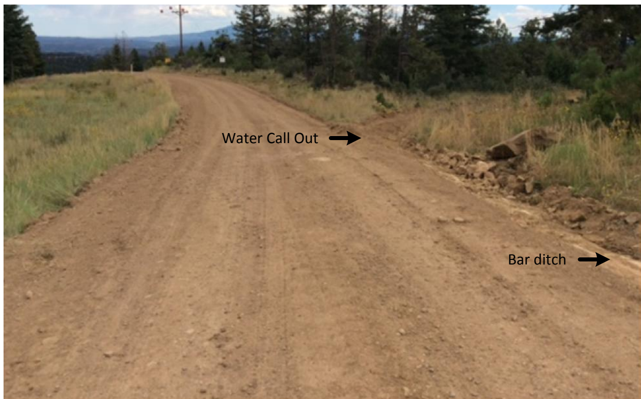
Photo 6: Facing east along the main access road, east of AC 02-14 well pad. Installed a water turn out to reduce the volume of run off flowing down the main road.
