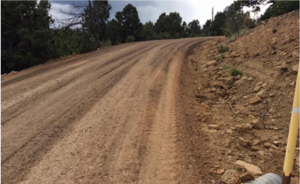
Photo 1: Facing west along the main road. Installed road base and crowned the driving surface to establish sheet flow. Dominated the bar ditch to receive run off.
