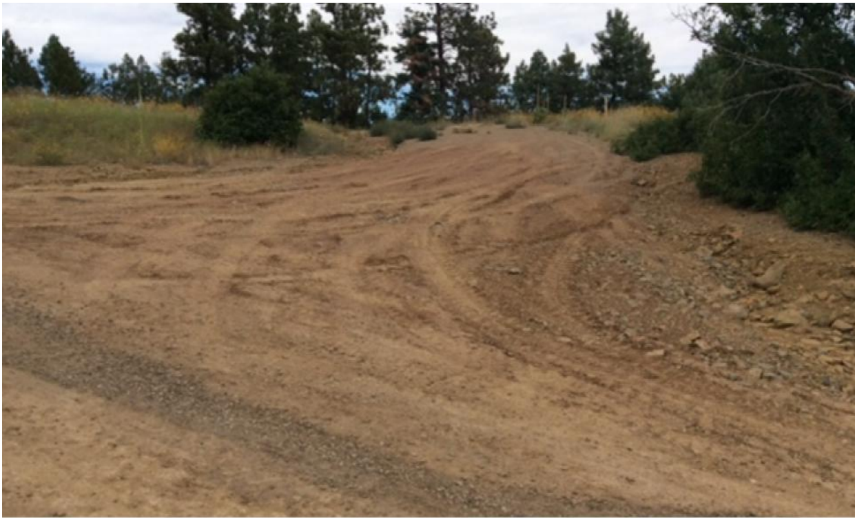
Photo 3: Facing northwest at the access road to AC 02-16V well pad. Installed road base and crowned the driving surface to establish sheet flow.
