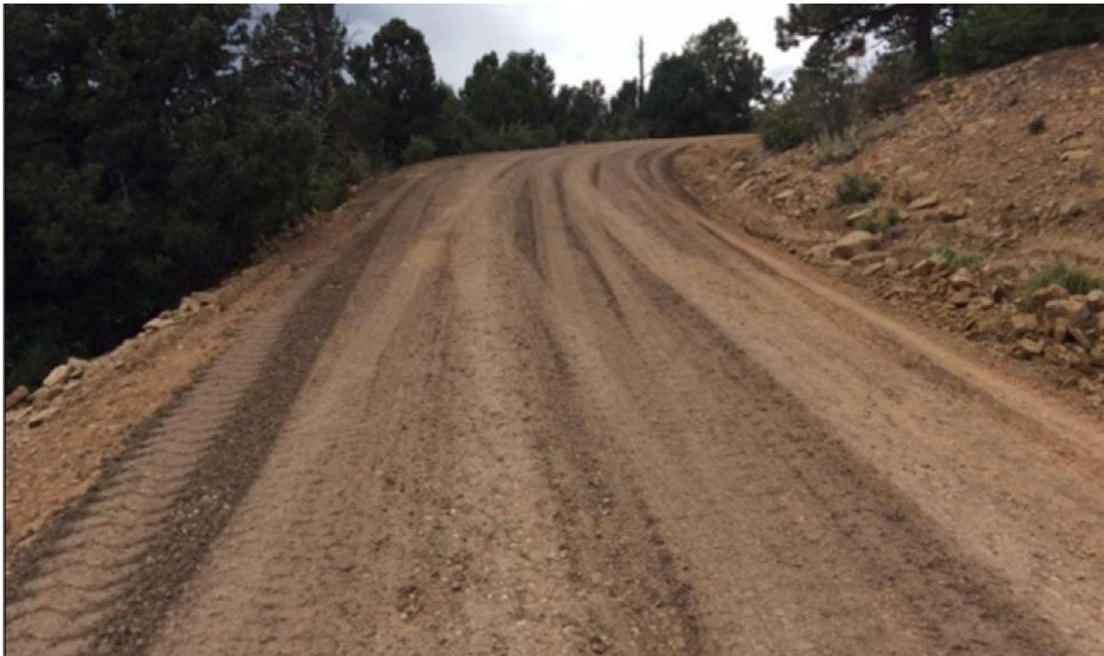
Photo 2: Surface crowning conveys sheet flow to both sides of the road, reducing the potential for surface erosion.
