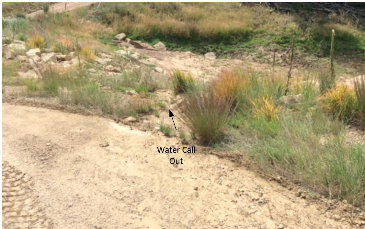
Photo 4: Access road to AC 01-12 well pad. Run off is diverted to an armored swell toward the culvert inlet.
