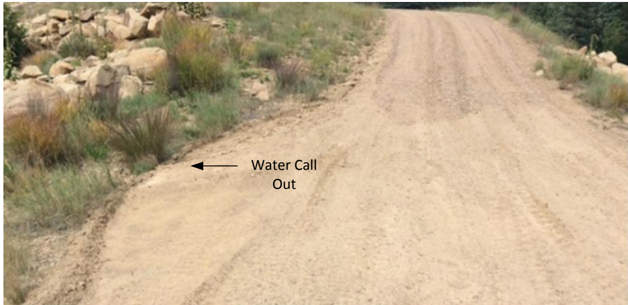
Photo 3: Access road to AC 01-12 well pad. Created a water call out to allow water to drain from the roadway surface to the west side of access road.
