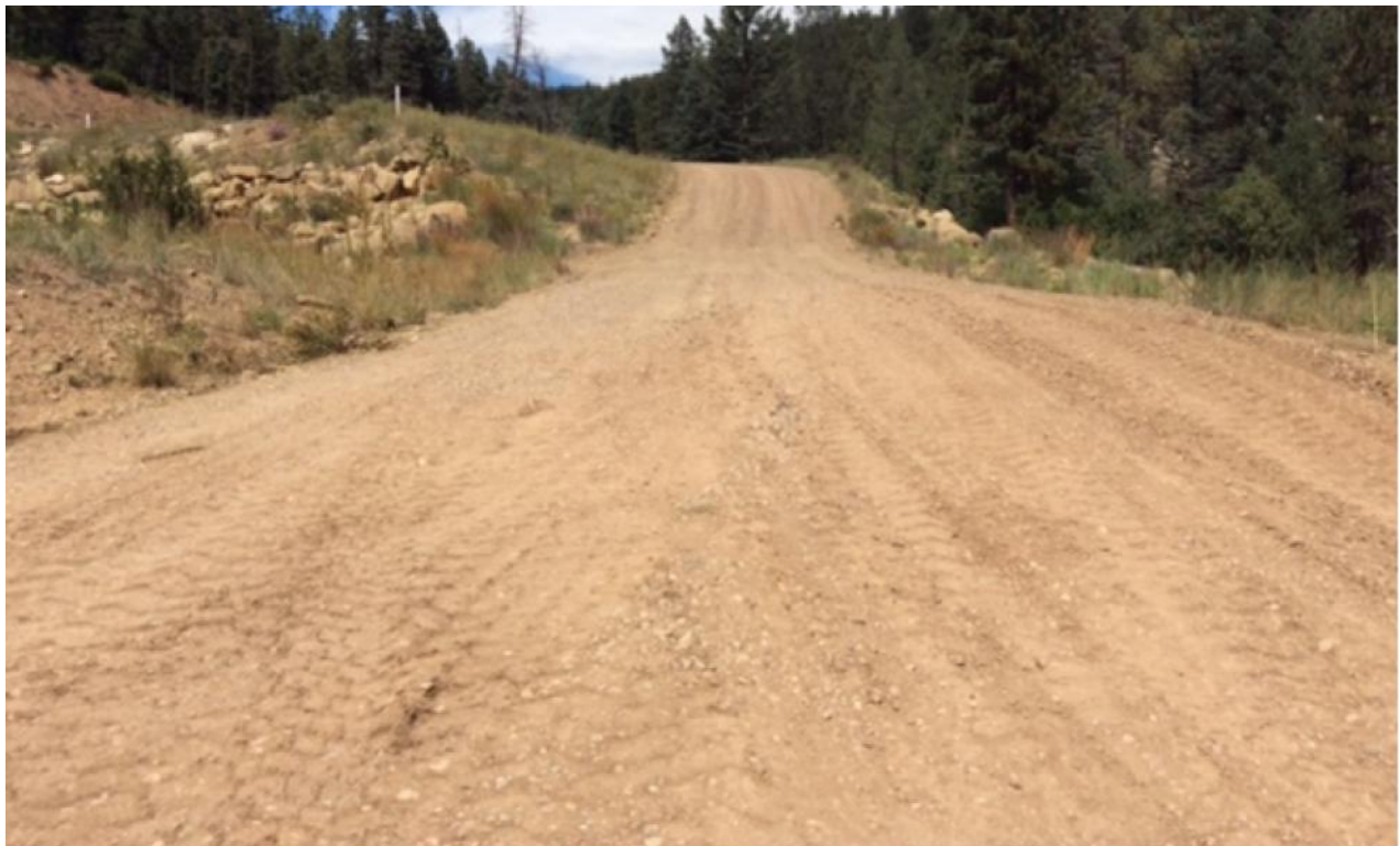
Photo 2: Access road to AC 01-12 well pad. Installed road base and surfaced crowned the driving surface to establish sheet flow.
