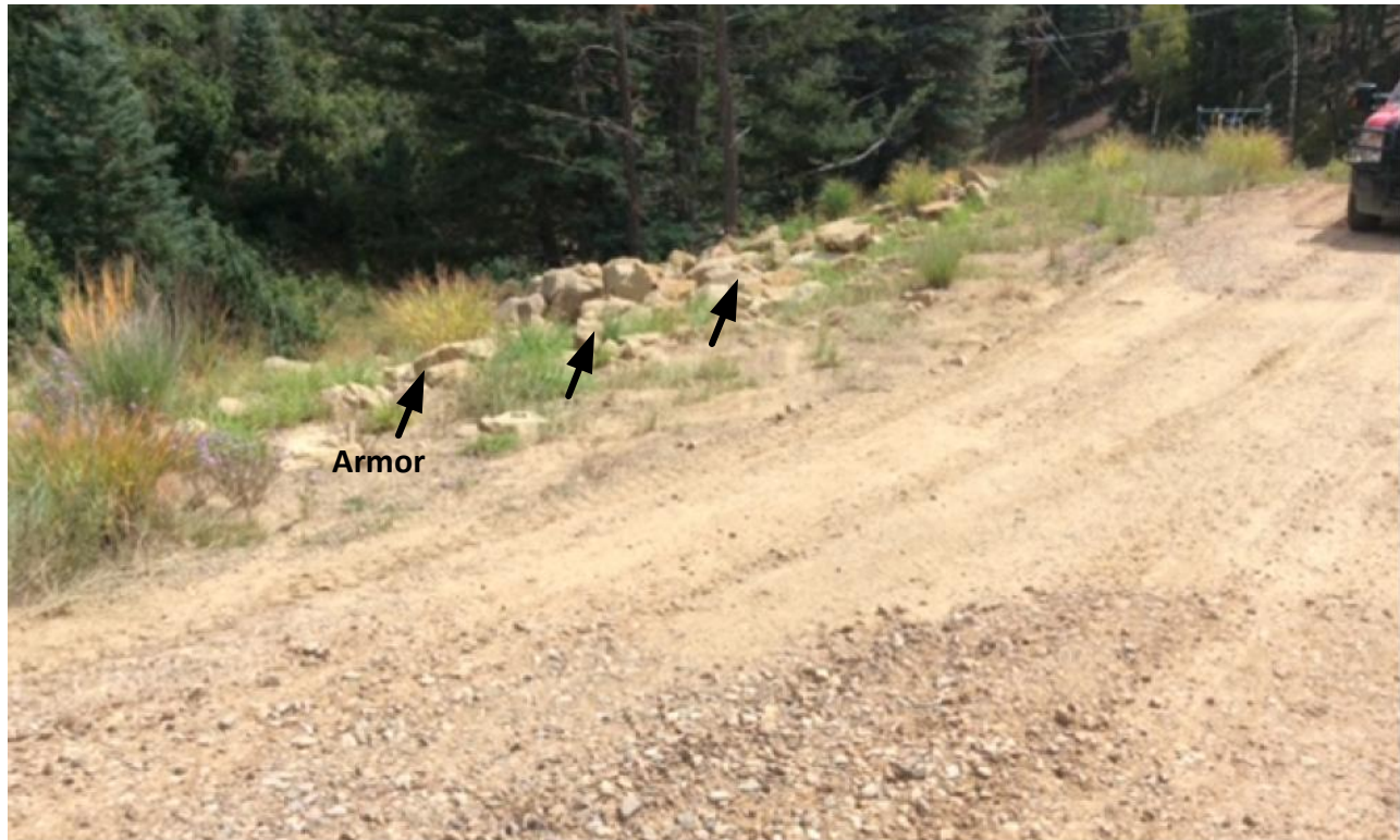
Photo 5: Access road to AC 01-12 well pad. Created sheet flow from the access road to drain water from the roadway surface to the east side of the access road where the existing armor on the culvert outlet side will be utilized for erosion control.
