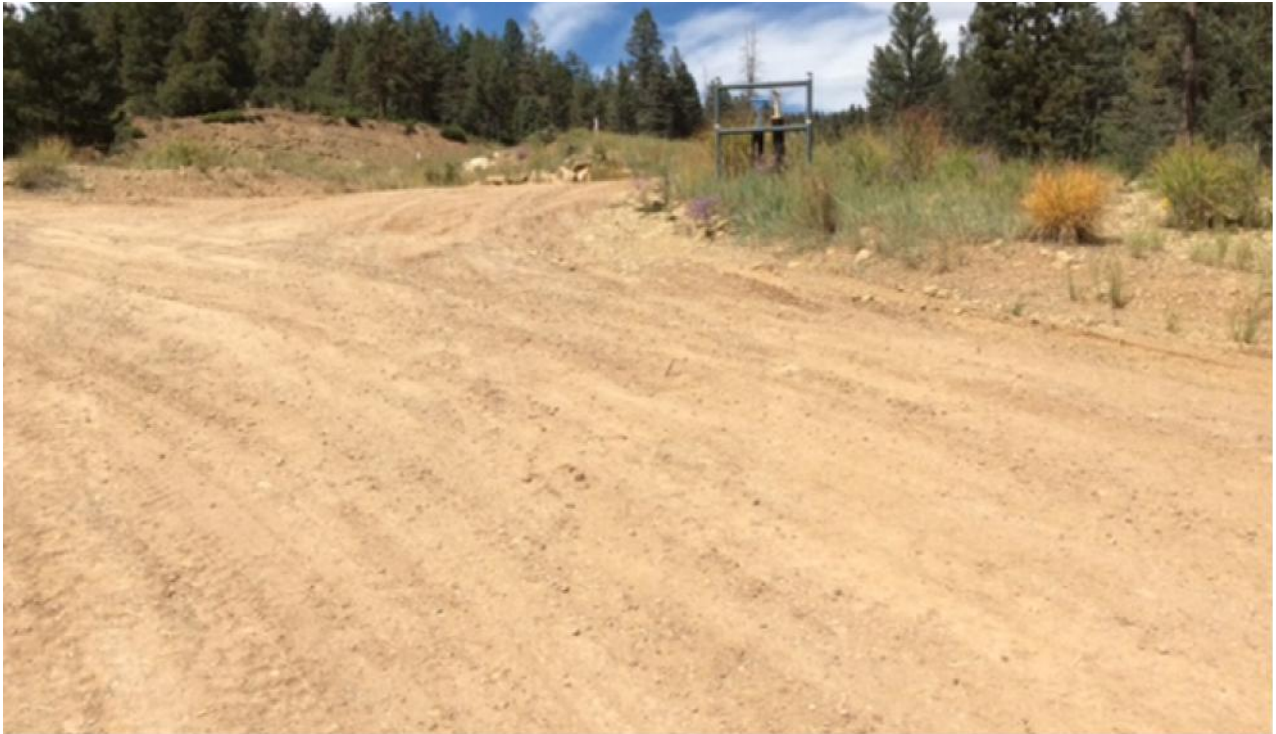
Photo 1: Facing west along the main road. Installed road base and surfaced crowned the driving surface to establish sheet flow.
