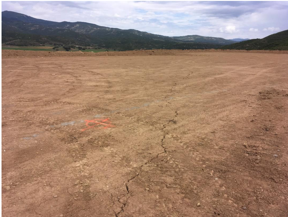
Photo No. 7 – Tension cracks in 24-7 pad looking NE.
