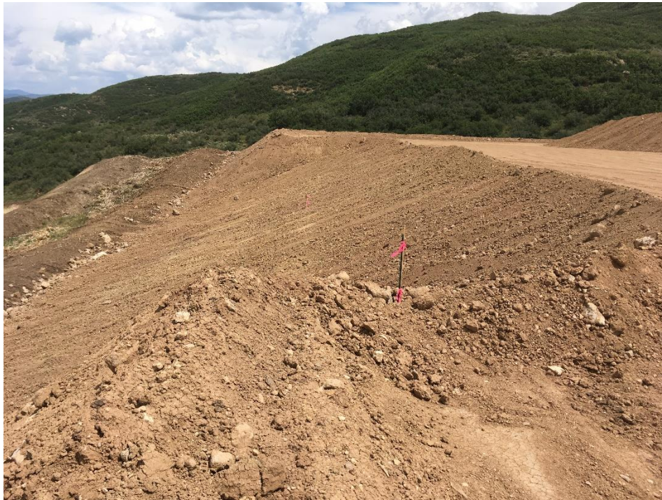
Photo No. 5 – Wedge of fill removed from N edge of 24-7 pad immediately following slope failure to remove driving force.
