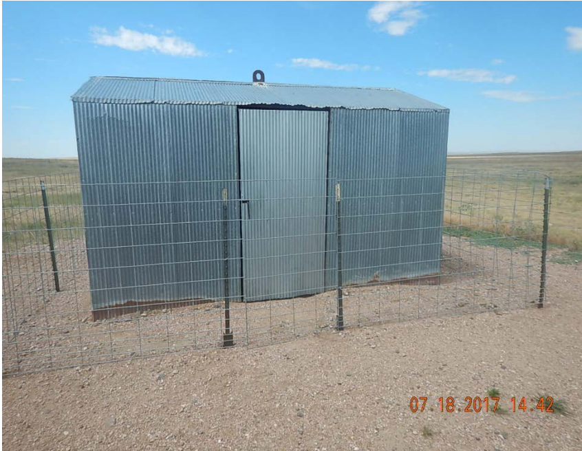
Photo 1: Wellhead, looking N
