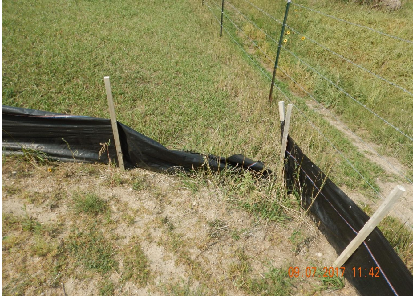
Photo 3. Photo taken from the southeastern location, facing South. BMP maintenance needed along a section of the silt fence.
