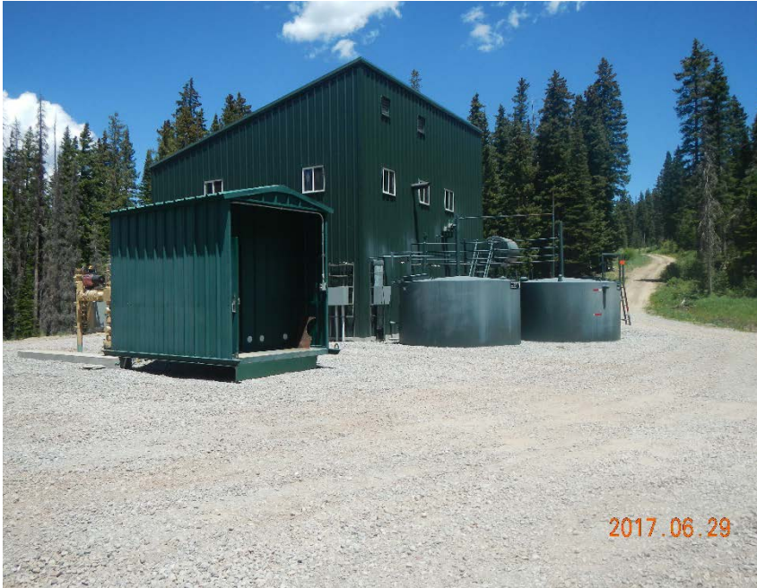
WC12 pad. Building and double wall tanks.
