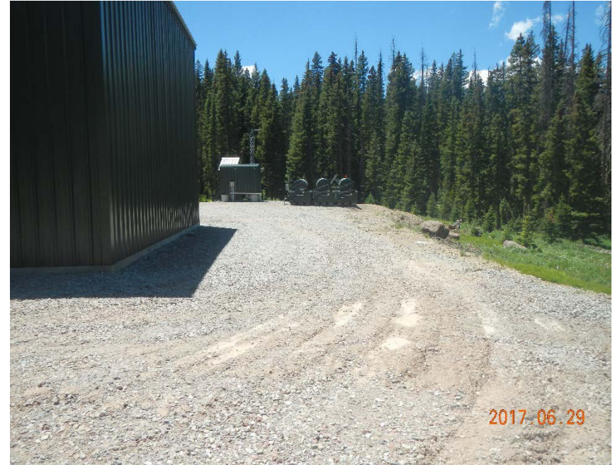
Back of building. Horizontal tanks in secondary containment. Berms on the perimeter of the pad .
