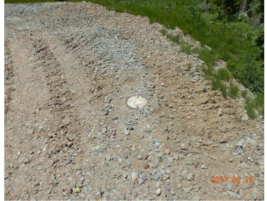
Flush-mount groundwater monitoring well on the pad.
