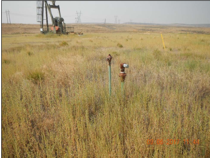
Photo 4. 1 -1" and 1 – 2" steel riser at 40.48676, - 107.81588
