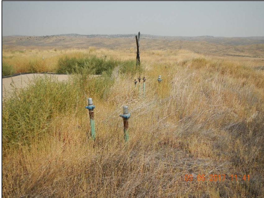
Photo 2. 3 – 2" and 3 – 1" steel risers at 40.48653, -107.81559
