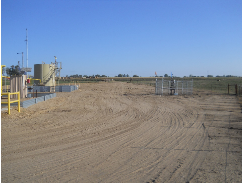
Southeast edge of location looking north. Erosion issues have been addressed. Weeds have been controlled
