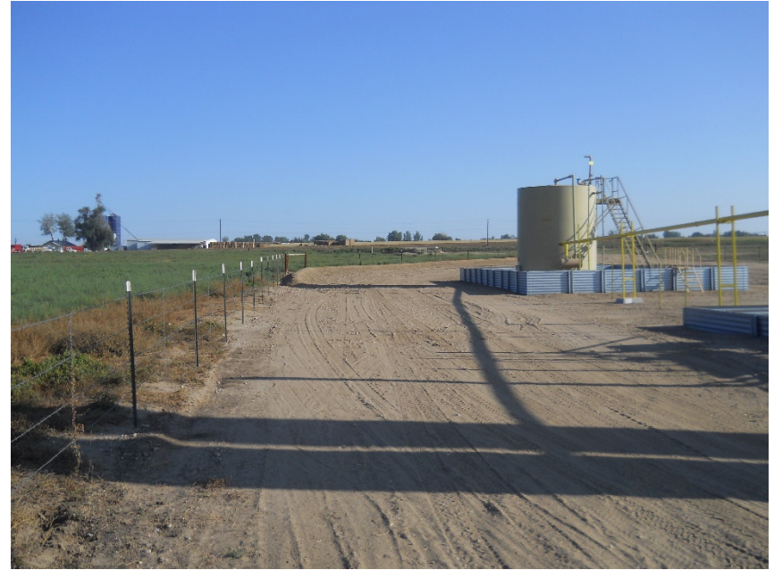
Southwest edge of location looking north. Erosion issues have been addressed, berm constructed on north/northwest edge of location
