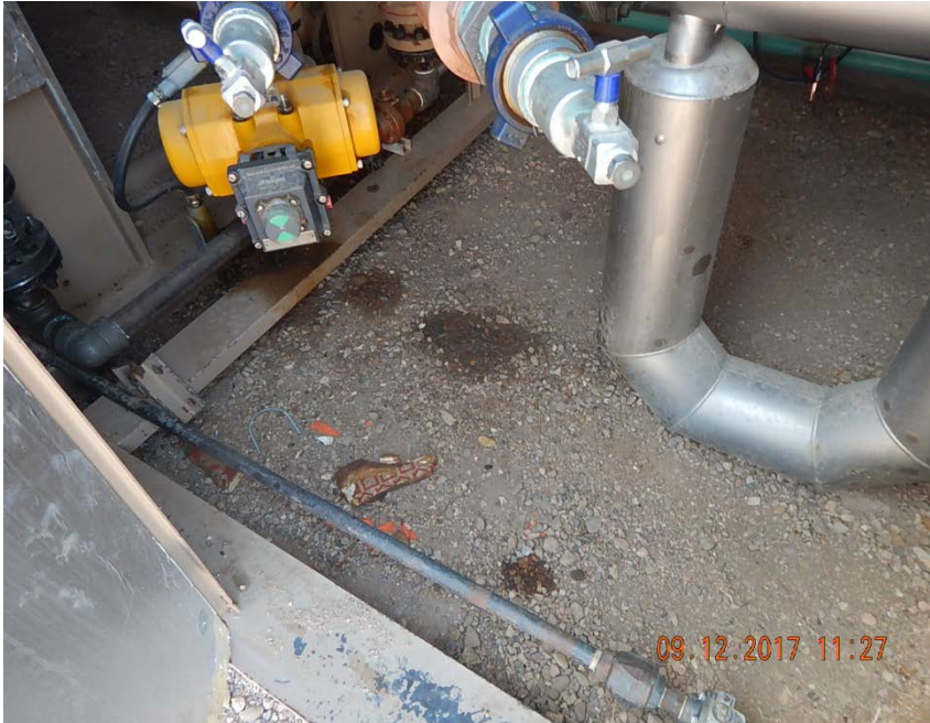
Photo 5: Stained soil in separator housing
