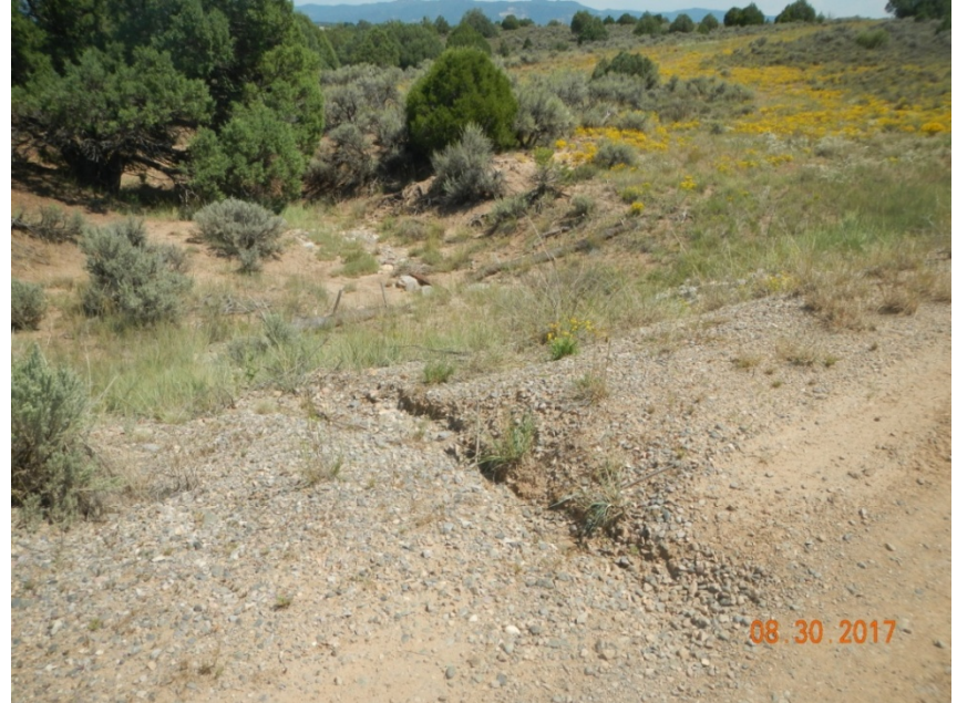
Photo 6: View of erosion occurring along the access road into a drainage. This area needs to be stabilized.
