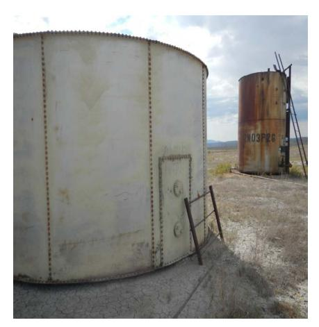
Photo#4: Staining, leak from pipe at base of Tank.
