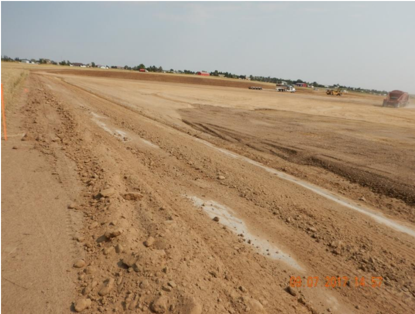
Photo 3. Photo taken from the northern location, facing East. Ditch BMP has been installed along the well pad perimeter.
