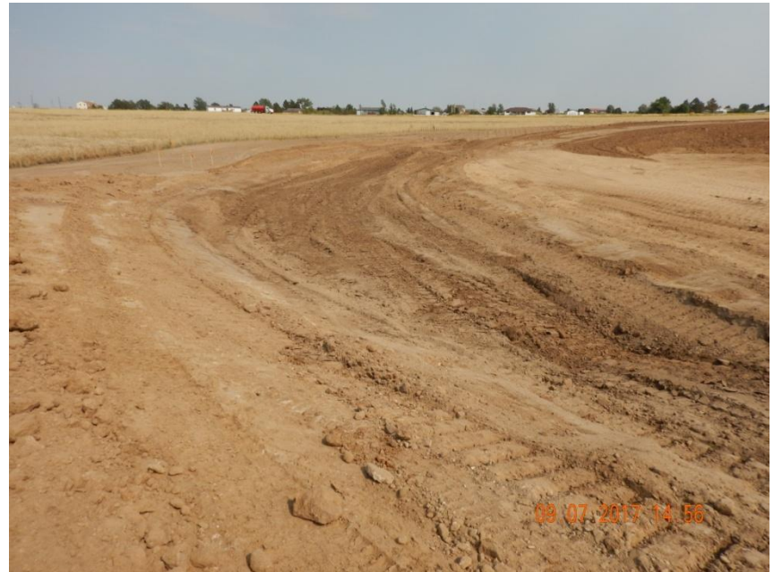
Photo 2. Photo taken from the northeastern location, facing East. Retention pond under construction for the permanent stormwater control BMP.
