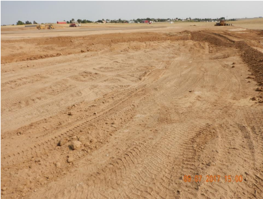
Photo 5. Photo taken from the southwestern location, facing Southeast. Retention pond under construction for the permanent stormwater control BMP.
