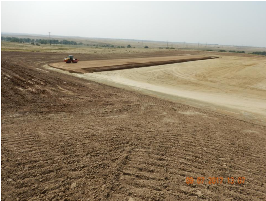
Photo 1. Photo taken from the eastern location, facing Southwest. Construction operations are still underway. Disturbance areas outside of the well pad have been temporarily stabilized with equipment.
