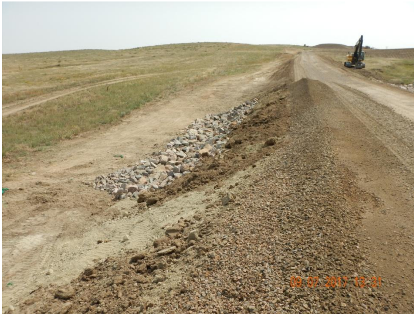
Photo 8. Photo taken from the east culvert area of the intermittent stream crossing, facing South. Operator In-Process of stabilizing culvert area. Operator shall ensure erosion and sediment controls are installed along access road portions to control and manage for sediment discharge.
