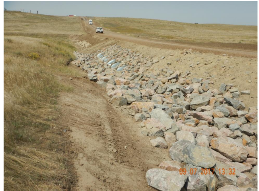
Photo 9. Photo taken from the west culvert area of the intermittent stream crossing, facing North. Operator In-Process of stabilizing culvert area. Operator shall ensure erosion and sediment controls are installed along access road portions to control and manage for sediment discharge.
