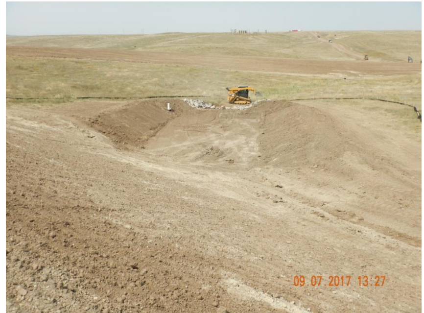
Photo 7. Photo taken from the northern location, facing North. Sediment trap construction underway.
