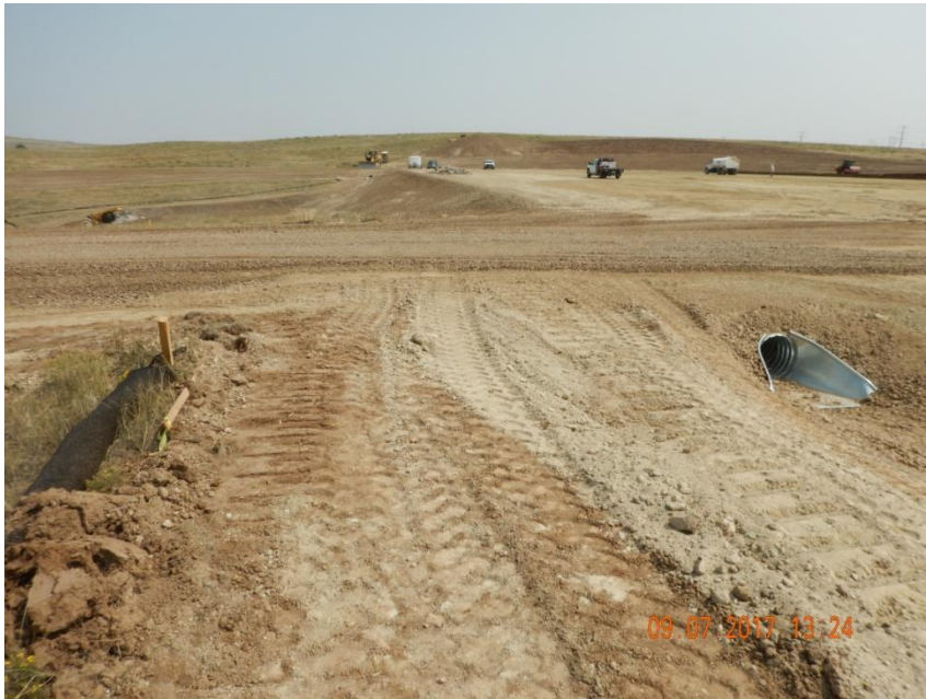
Photo 6. Photo taken from the northern well pad, west access entrance to location, facing East. Culvert installed with a stabilized outlet area. Culvert installed in conjunction with the well pad perimeter ditch. Stormwater runoff is being directed to a sediment trap-see photo 7.
