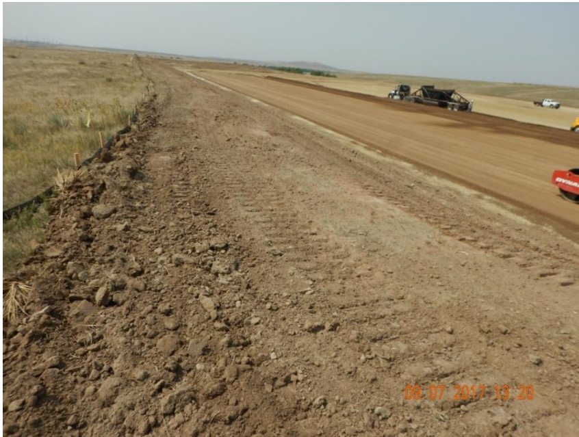
Photo 4. Photo taken from the southern location, facing West. Temporary Filtrexx BMP installed around the southern location. Cut slopes have been temporarily stabilized. It should be noted that equipment did not correctly track some cut slopes such that the grooves run perpendicular to the cut slopes. Operator will mulch and seed all disturbance area outside of the well pad. Perimeter ditch around well pad.
