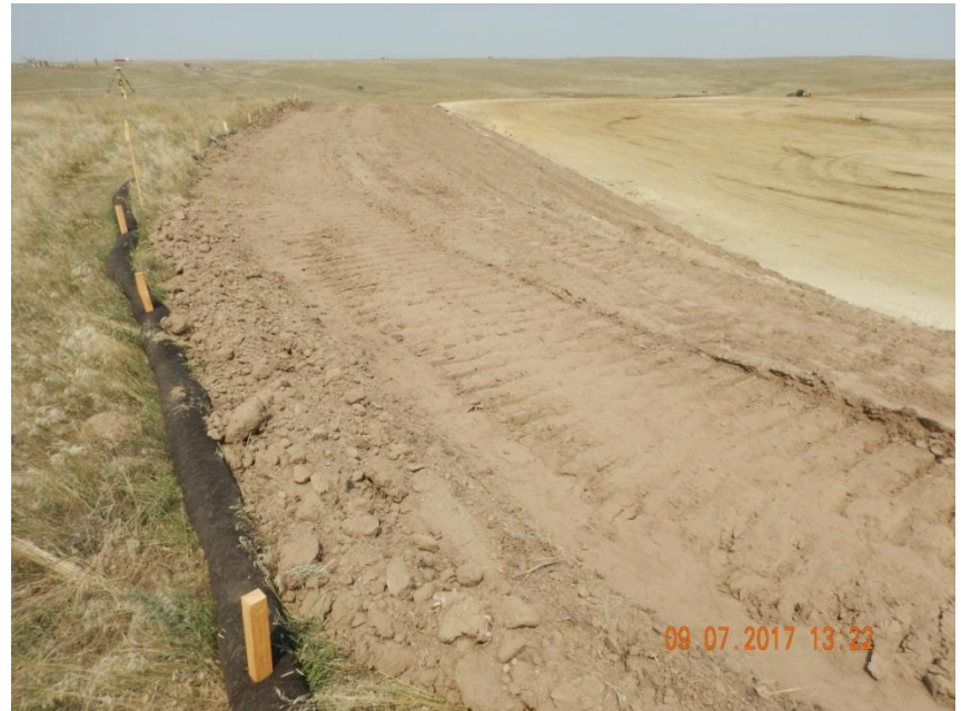
Photo 5. Photo taken from the western location, facing North. Temporary Filtrexx BMP installed around portions of the western location. Perimeter ditch around well pad.
