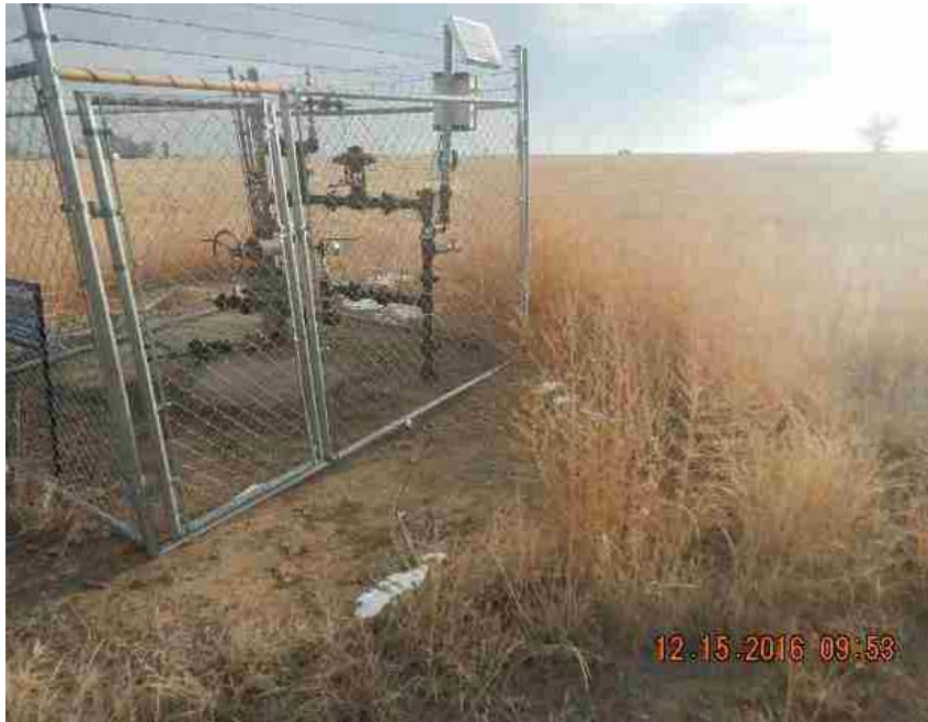
Photo from prior inspection for comparison
