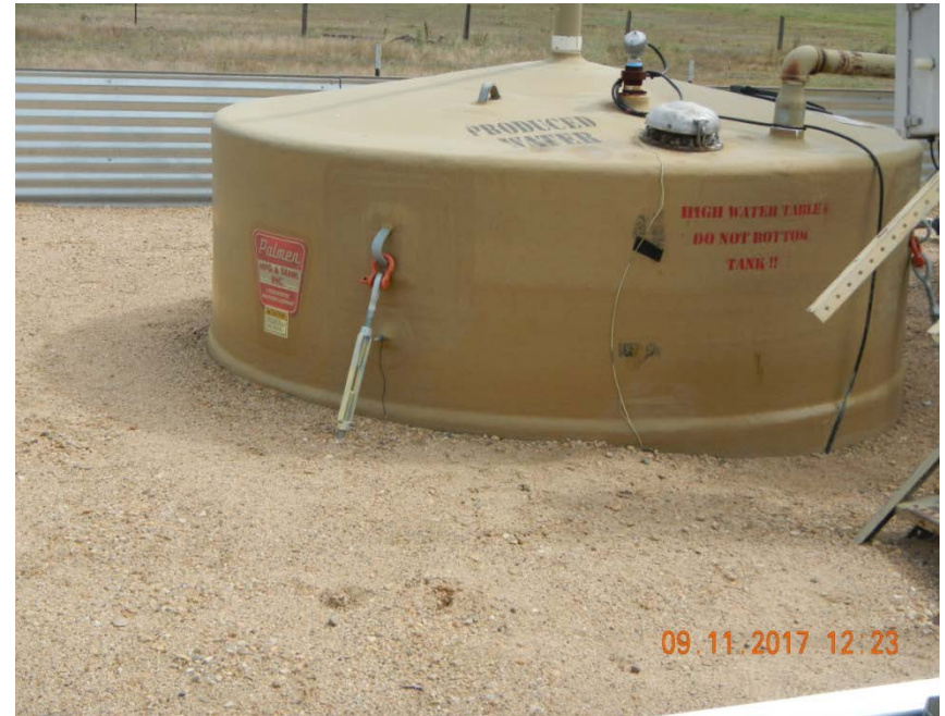
Produced water vault anchors
