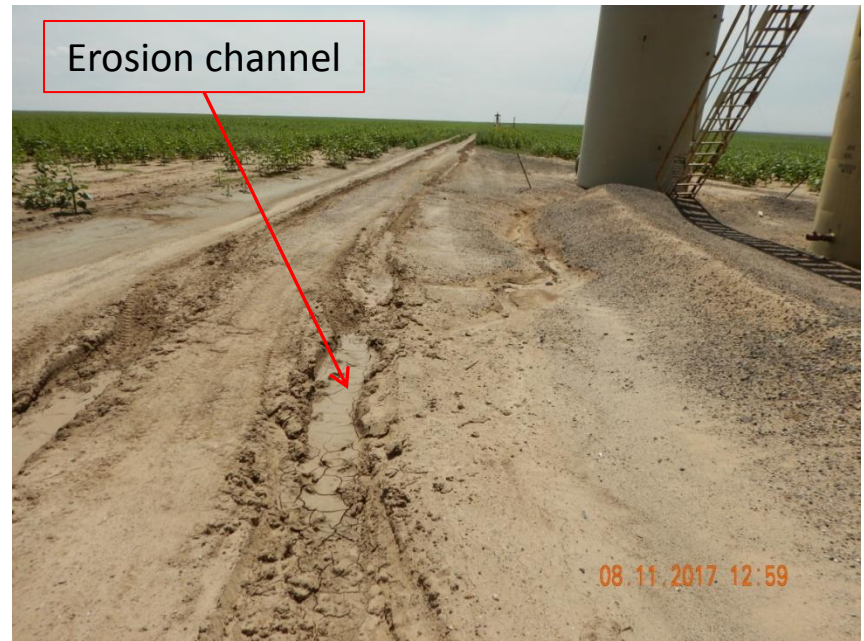
Photo 2. Photo taken August 11, 2017 from the previous photo location, facing South. Stormwater erosion evident as an erosion channel funnels around the northern battery location and continues off location into the adjacent cropland.
