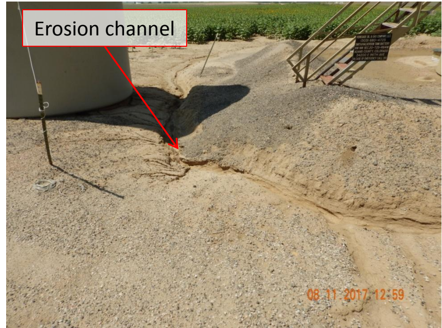
Photo 4. Photo taken August 11, 2017 from the previous photo location, facing West. Gully erosion observed from the previous inspection.
