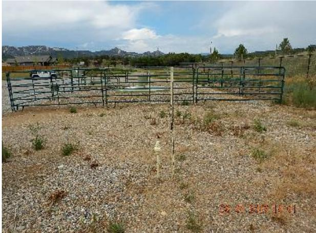
**Photo 7: 1" riser to the right of production tank behind power panel. Valve not tagged or locked out.**
