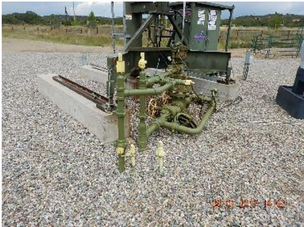
**Photo 9: Two 1" risers at wellhead. Valve not tagged or locked out. Previous inspection.**
