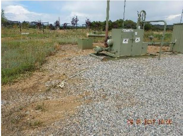
**Photo 3: Downed anchor marker. Previous inspection.**
