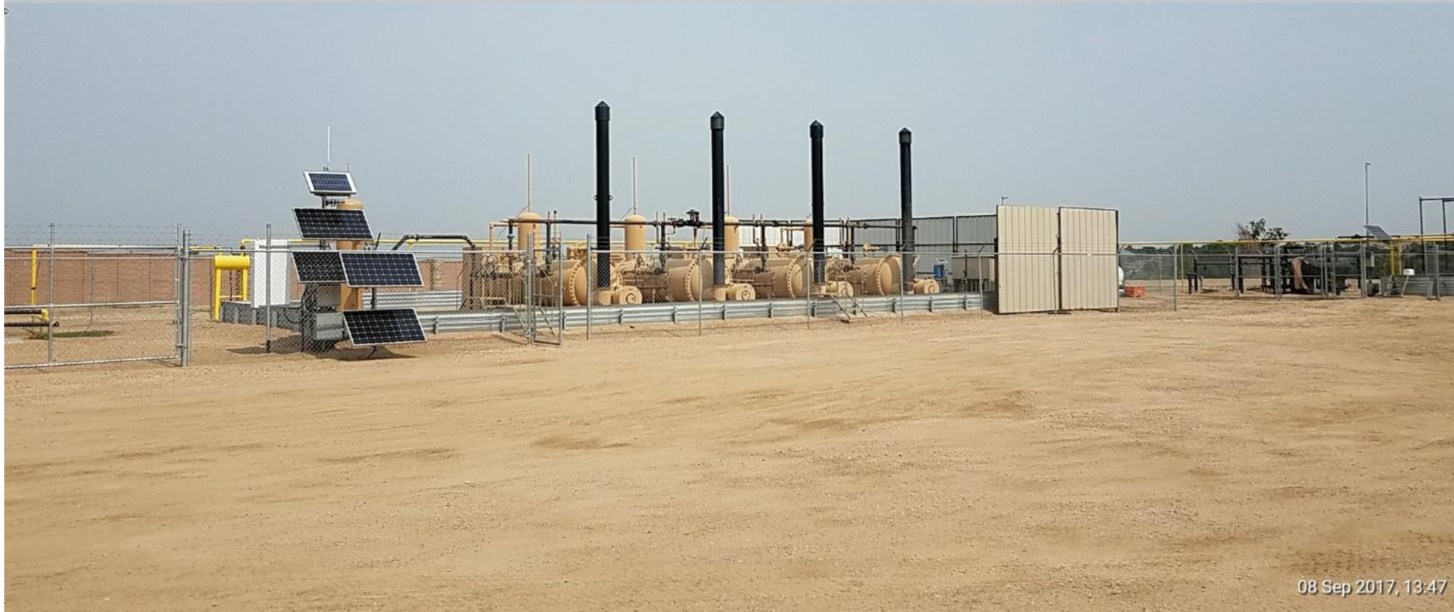
Heated horizontal separators and small compressors.
