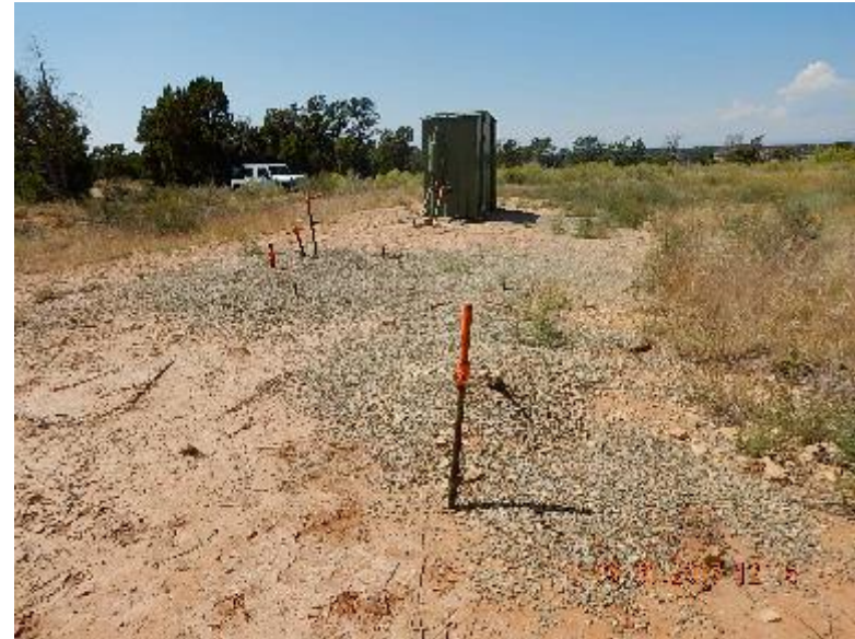
Photo 4: (4) risers off backside of gas meter run shed.
