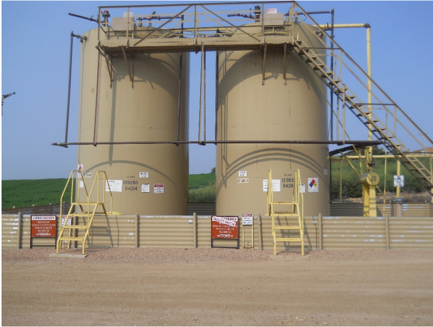
Tank battery looking west
