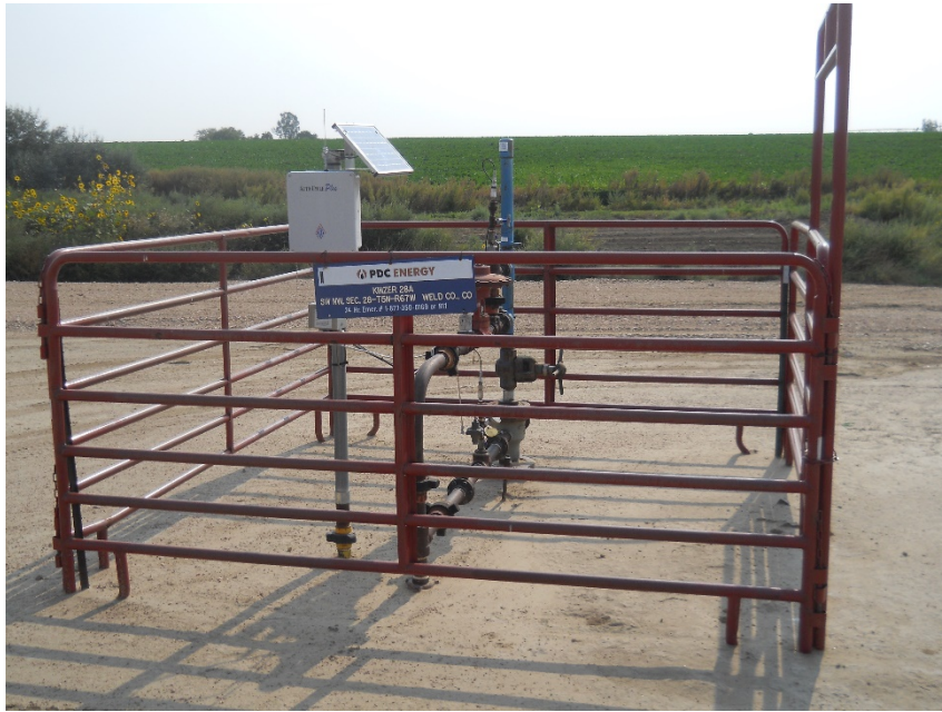
Kinzer 28A wellhead looking east
