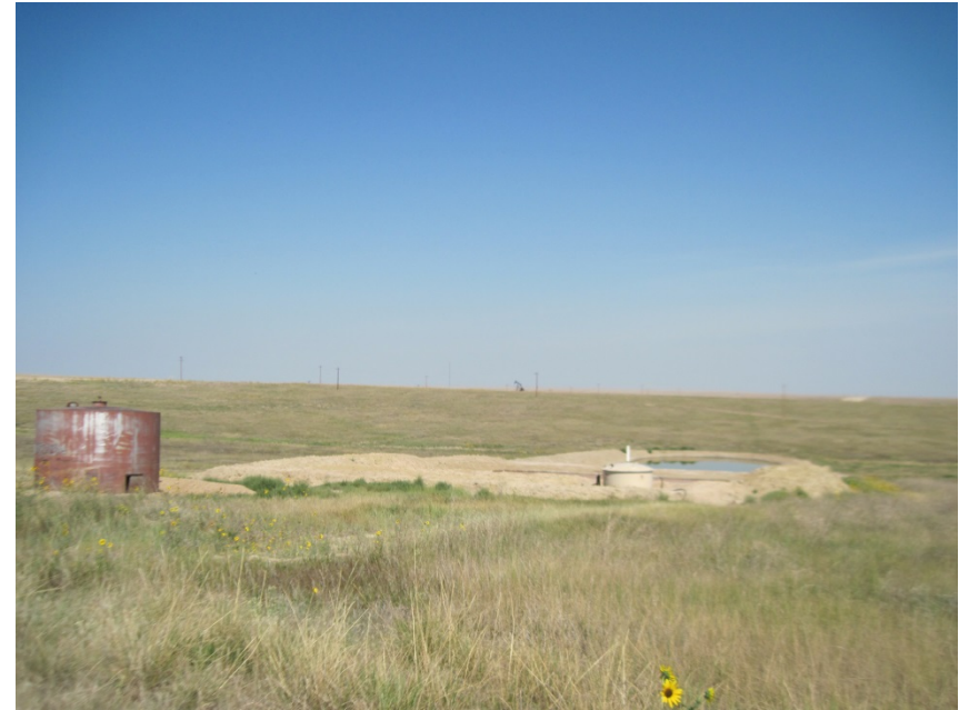
UNUSED METAL TANK AND PITS
