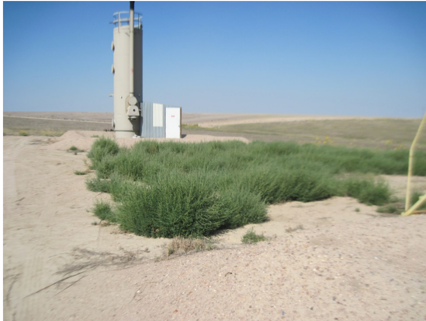
WEEDS ON BATTERY LOCATION
