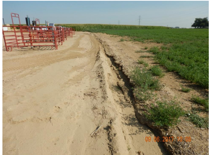
Photo 2. Photo taken September 6, 2017 from the northeast location, facing North. Appears the Operator has built up a berm along the north and northeast location to divert run-on onto location through an eastern ditch.
