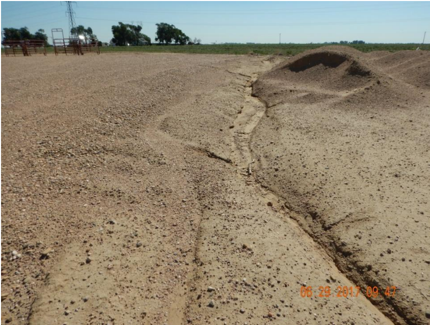
Photo 3. Photo taken on June 29, 2017 from the southern location, facing East. Gully erosion is occurring adjacent to the location from stormwater and/or irrigation water run-on onto location.
