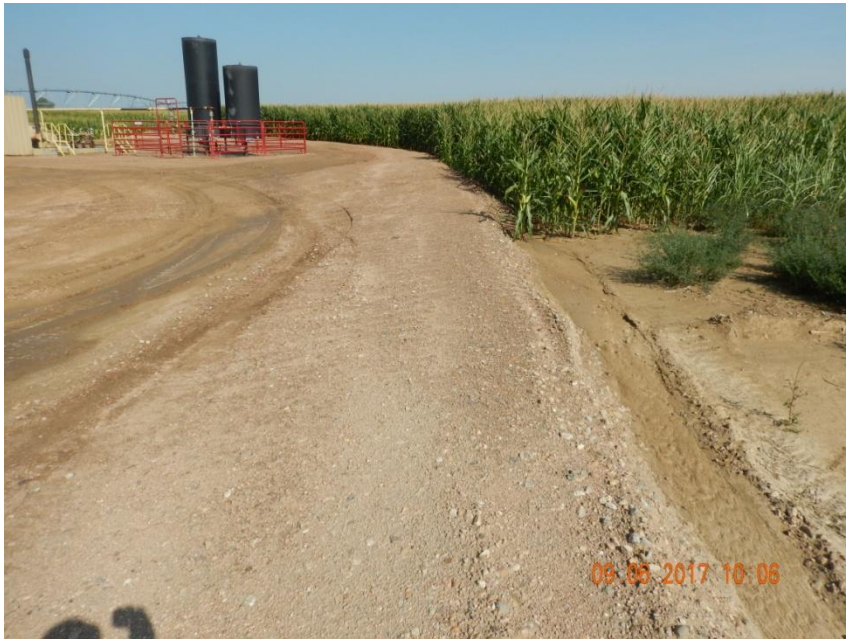
Photo 5. Photo taken on September 6, 2017 from the northeast location, facing North. Photo illustrates berm that has been built to divert run-on onto location.
