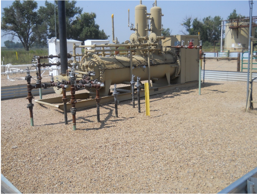
3-2" steel marked active risers east side of separator
