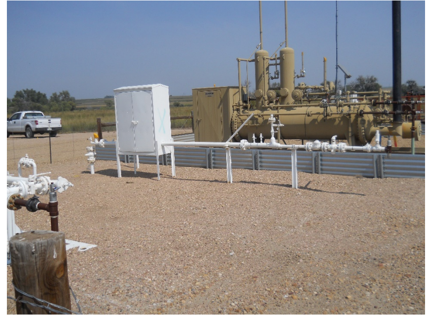
Unused disconnected meter run west of separator
