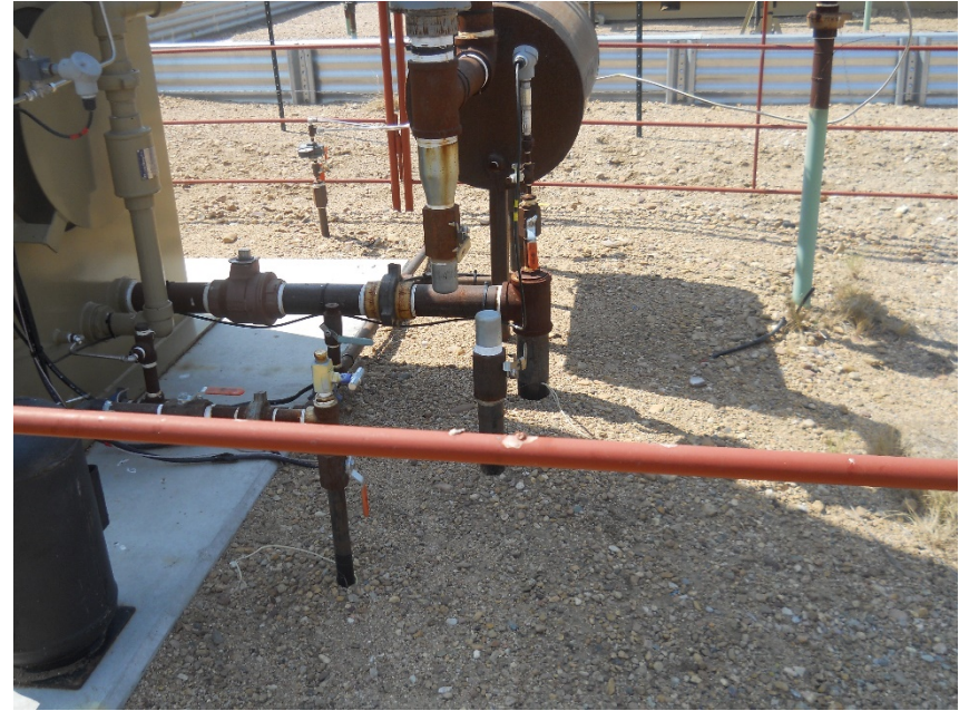
2" steel marked active riser north side of ECD
