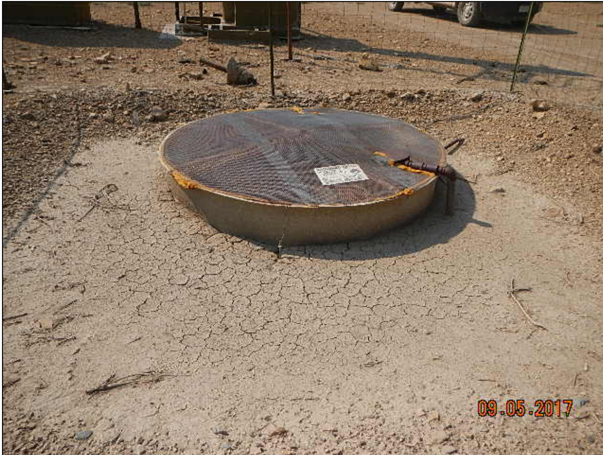
Photo 1. Sign is faded and capacity not listed.
