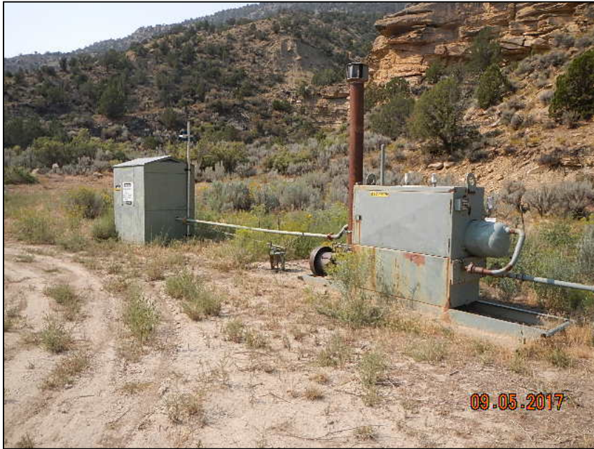
Photo 1. Vegetation around equipment.
