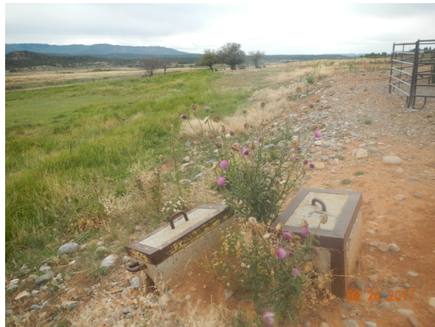
Photo 4: View of the eastern portion of the project area facing southward. Unused anchors in foreground do not appear needed.
