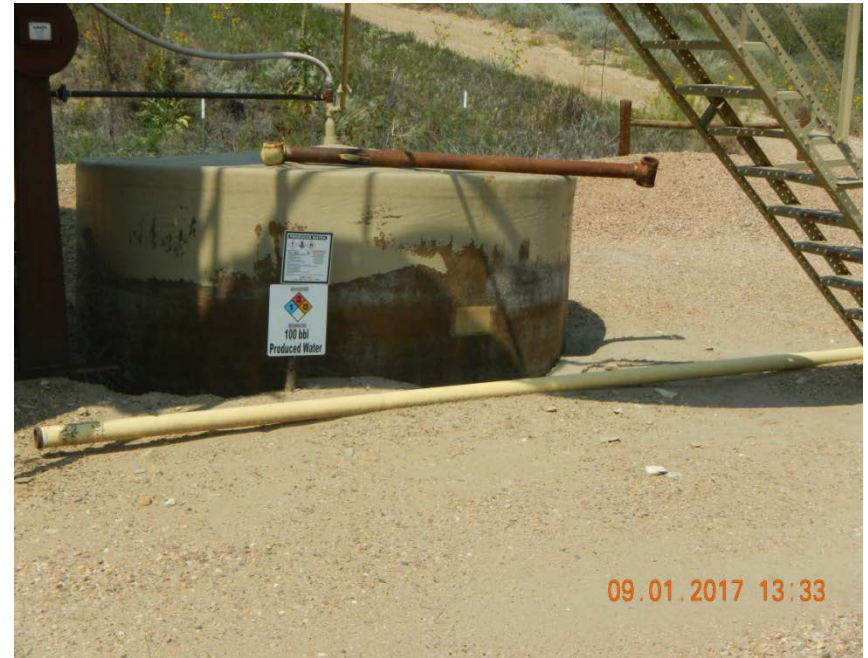
Unused load line
