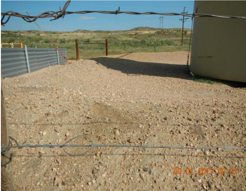
Crude oil tank berm
