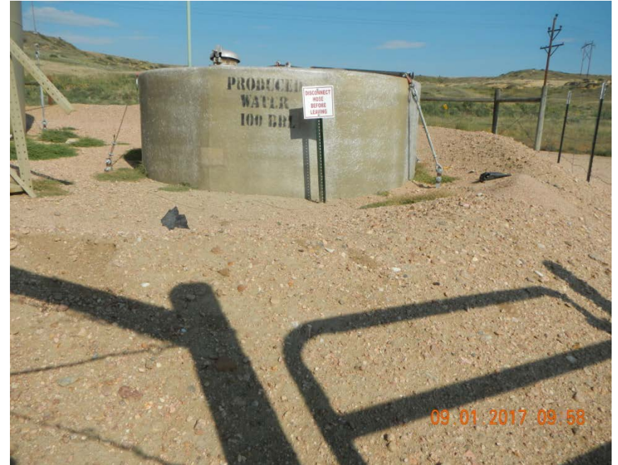
Crude oil tank berm
