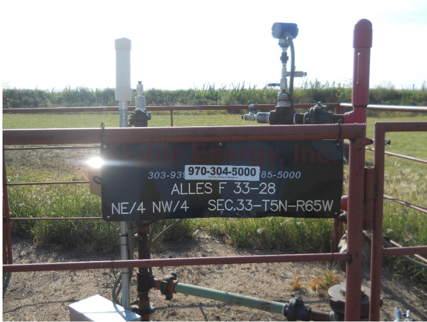
Wellhead sign looking east
