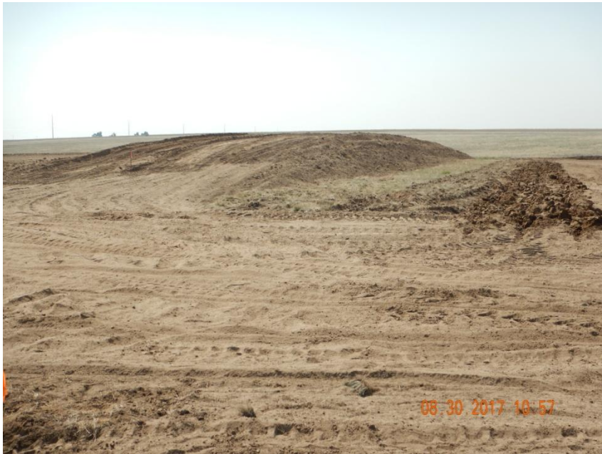
Photo 3. Photo taken from the central location, facing South. Appears Operator has salvaged and stored topsoil along the central location.
