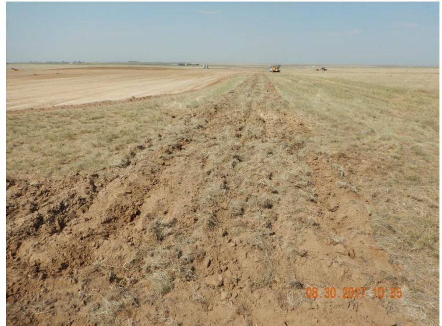
Photo 2. Photo taken from the northeast location, facing West. Operator has installed surface roughening around the perimeter of the location.
