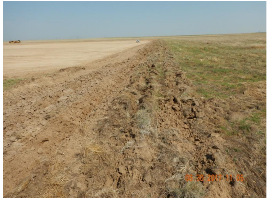
Photo 6. Photo taken from the southeast location, facing North. Operator has installed surface roughening around the perimeter of the location.
