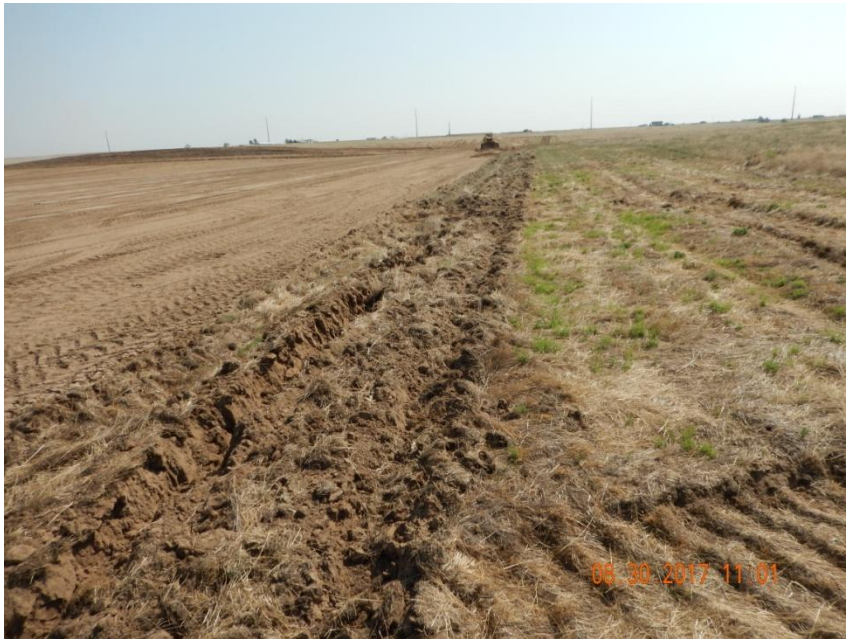
Photo 5. Photo taken from the southwest location, facing East. Appears Operator has salvaged and stored topsoil along the central location.
