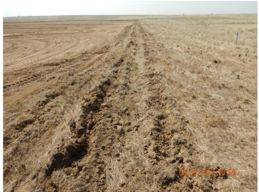
Photo 4. Photo taken from the northwest location, facing South. Operator has installed surface roughening around the perimeter of the location.
