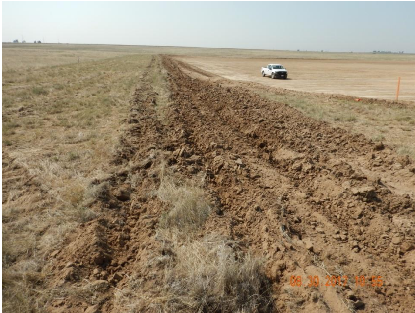
Photo 1. Photo taken from the northeast location, facing South. Operator has installed surface roughening around the perimeter of the location.
