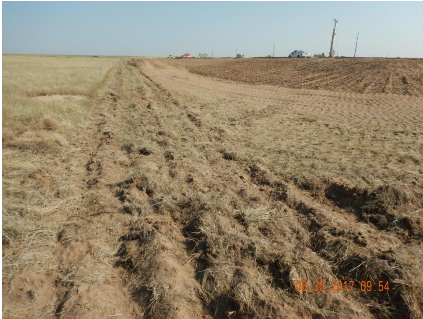
Photo 1. Photo taken from the southwest location, facing North. Operator has installed surface roughening around the perimeter of the location. Fill slopes appear to be temporarily stabilized.
