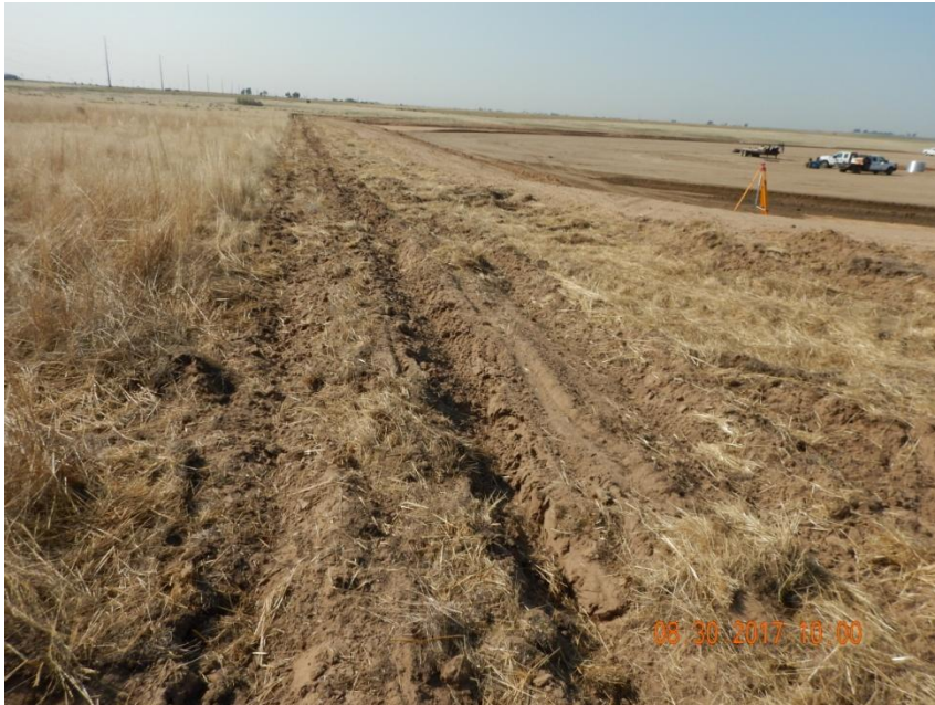
Photo 3. Photo taken from the northeast location, facing South. Operator has installed surface roughening around the perimeter of the location.
