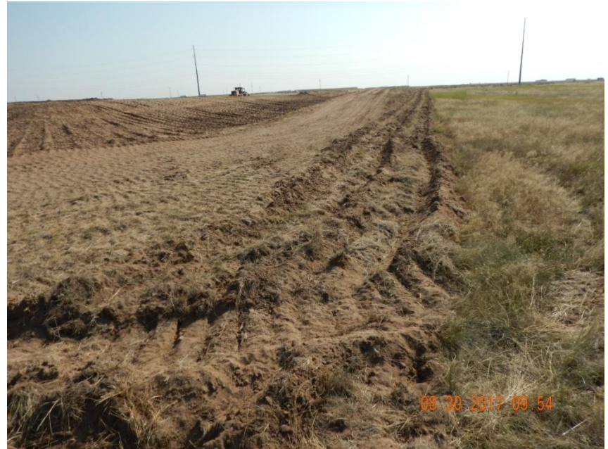
Photo 2. Photo taken from the southwest location, facing North. Operator has installed surface roughening around the perimeter of the location. Fill slopes appear to be temporarily stabilized.
