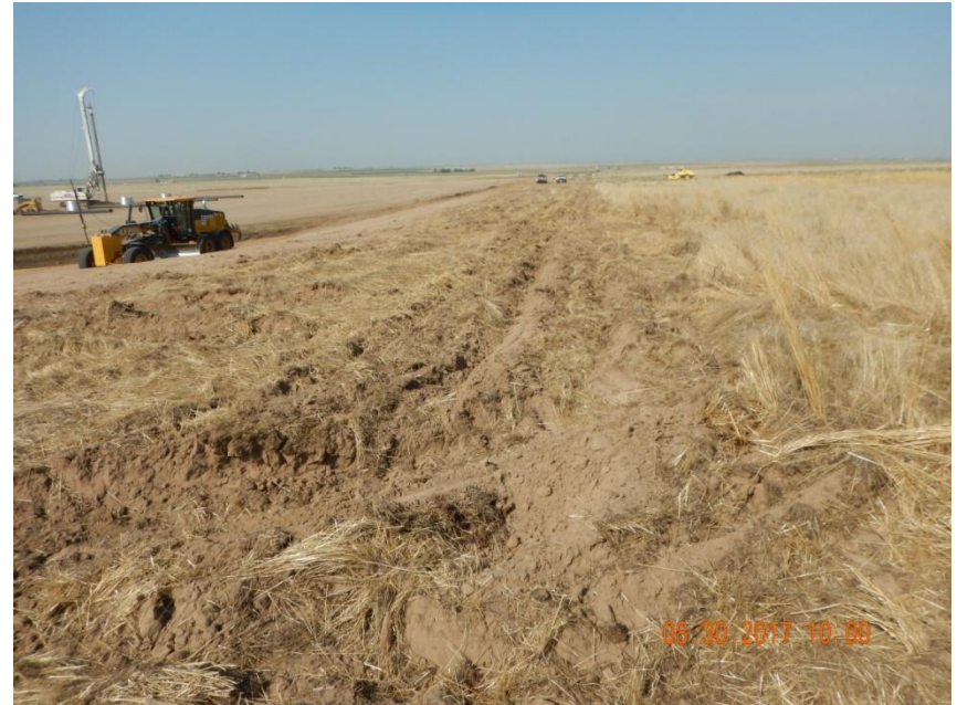
Photo 4. Photo taken from the northeast location, facing West. Operator has installed surface roughening around the perimeter of the location.
