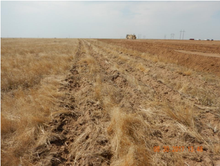
Photo 3. Photo taken from the southeast location, facing West. Operator has installed surface roughening around the perimeter of the location.
