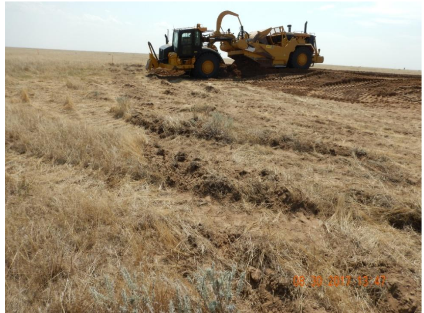
Photo 2. Photo taken from the southeast location, facing South. Operator has installed surface roughening around the perimeter of the location. Equipment traffic (tractor-scraper) traveling over BMP. BMPs need to be maintained to ensure the BMP is properly functioning.
