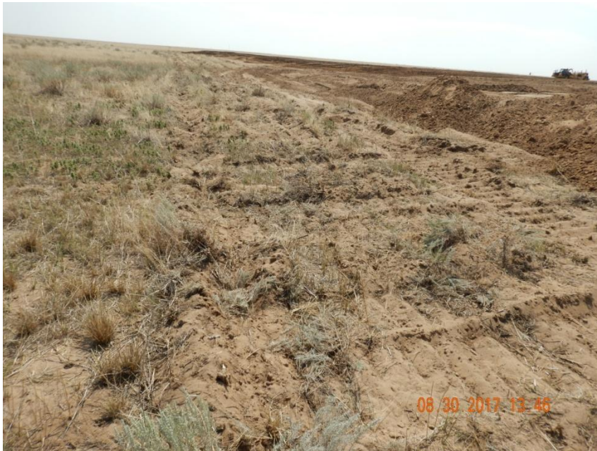
Photo 1. Photo taken from the northeast location, facing South. Operator has installed surface roughening around the perimeter of the location. Equipment traffic appears to have traveled over the BMP. BMPs need to be maintained to ensure the BMP is properly functioning.
