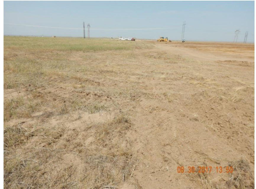
Photo 4. Photo taken from the southwest location, facing North. Operator has installed surface roughening around the perimeter of the location. Equipment traffic appears to have traveled over the BMP. BMPs need to be maintained to ensure the BMP is properly functioning.
