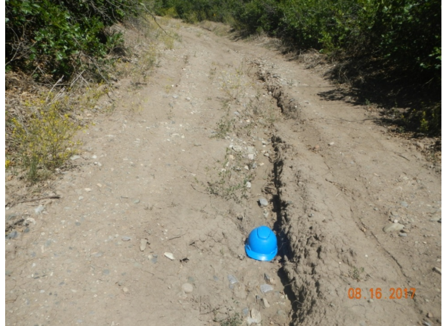
Photo 4: View of erosive channel occurring along the access road, approximately 1 foot wide and deep within the access road.
