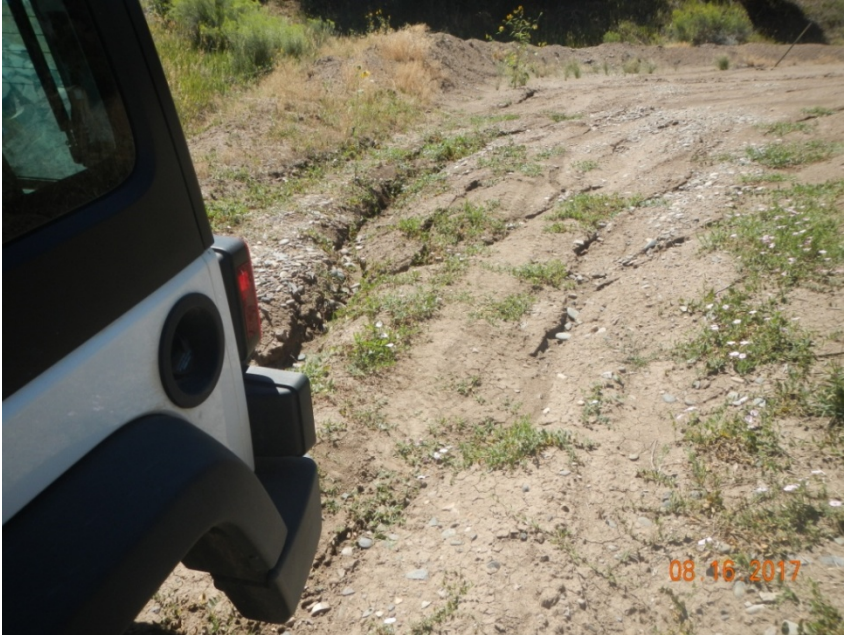
Photo 5: View of erosional channel on the access road near the well pad entrance.
