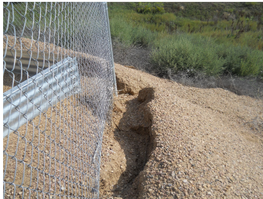
Erosion southeast corner of separator. Operator was contacted, construction crew in process of installing BMP's
