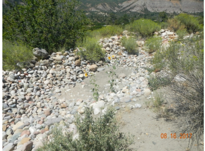
Photo 4: View of cobble-armored silt trap in the southern portion of the project area.
