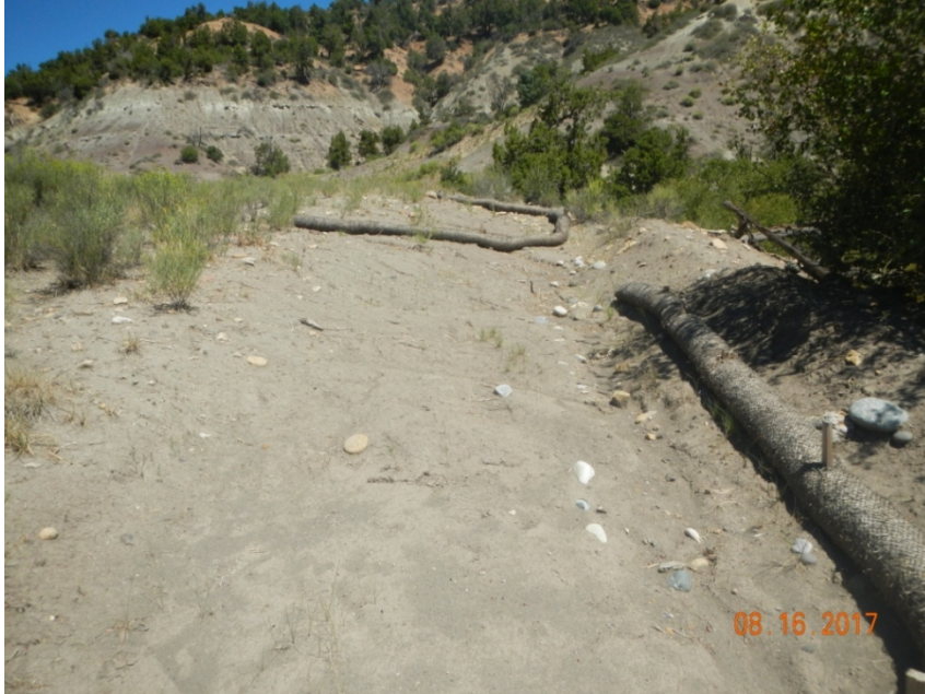
Photo 3: View of wattles where stormwater flows down the southeastern portion of the project area.
