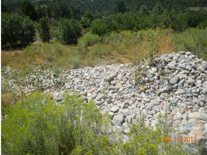
Photo 5: View of newly armored cobble-overflow channel in silt trap in the southern portion of the project area.
