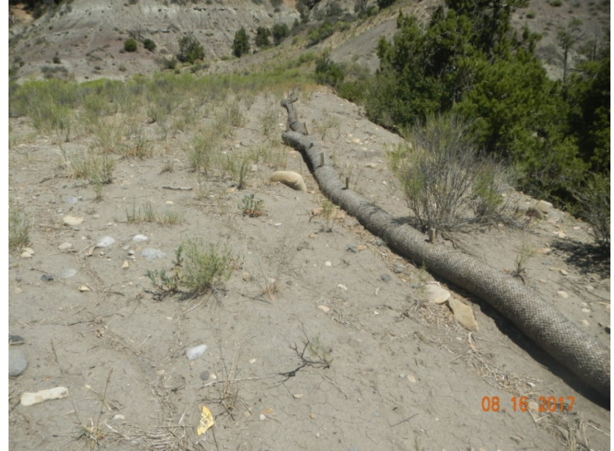
Photo 2: View of straw wattles placed along the eastern edge of the well pad, appear to be functioning at this time.
