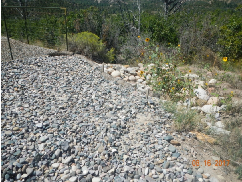
Photo 1: View of area documented in previous inspection with erosive channel, that is armored and stabilized at this time.
