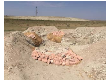
Sediment trap with inlet and outlet protection
