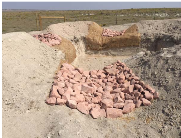
Sediment trap with inlet and outlet protection
