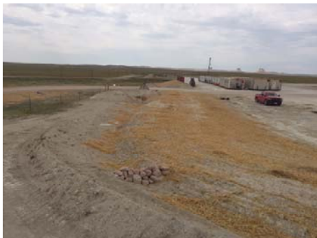
Perimeter Diversion Ditch with velocity check
