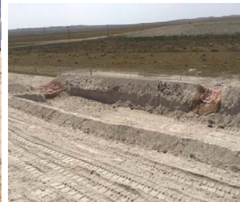
Sediment trap with inlet and outlet protection
