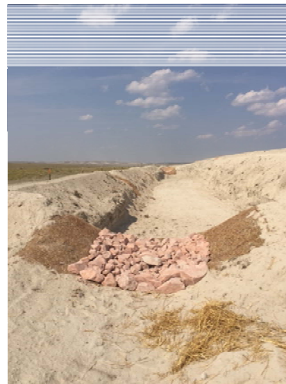
Sediment trap with inlet and outlet protection
