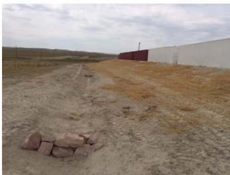
Perimeter Diversion Ditch with velocity check
