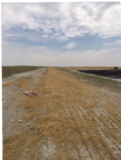
Perimeter Diversion Ditch with velocity check
