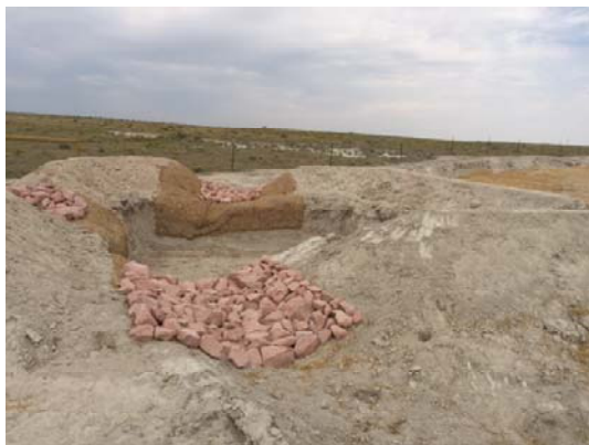
Sediment trap with inlet and outlet protection
