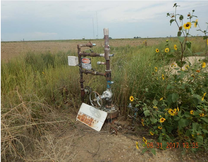
Photo 1: Wellhead, looking N. No bradenhead at surface, weeds around wellhead.
