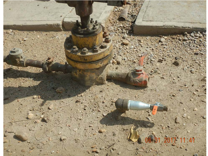
Photo 1: Stained soil removed, bradenhead plumbed to surface
