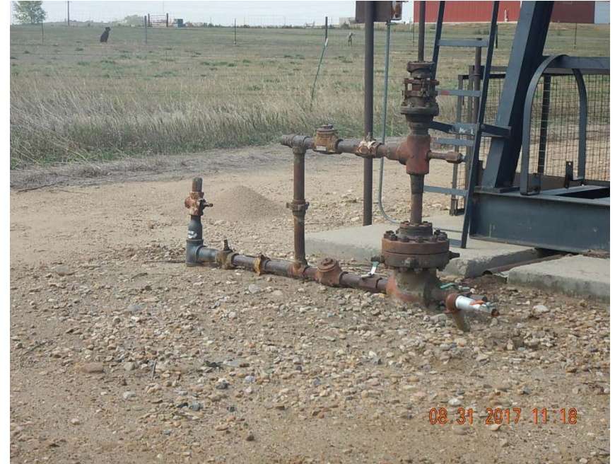
Photo 1: Fence removed, bradenhead plumbed to surface.
