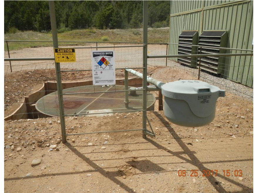
Drip pot on load out line.
