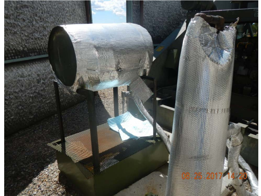
Lube oil container with secondary containment.
